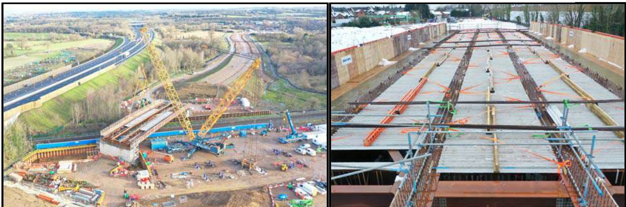
Figure 29: Typical example of lifting operation for installation of bridge beams and completed GRP Panels and Cantilever Formwork
