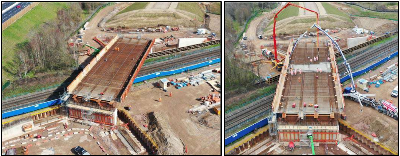
Figure 30: Typical example of lifting operation for installation of bridge beams and completed GRP Panels and Cantilever Formwork
