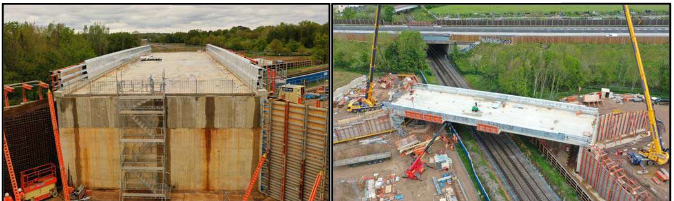
Figure 31: Typical example of lifting operation for installation of Parapet Fencing and the removal of the Cantilever Paraslim Units
