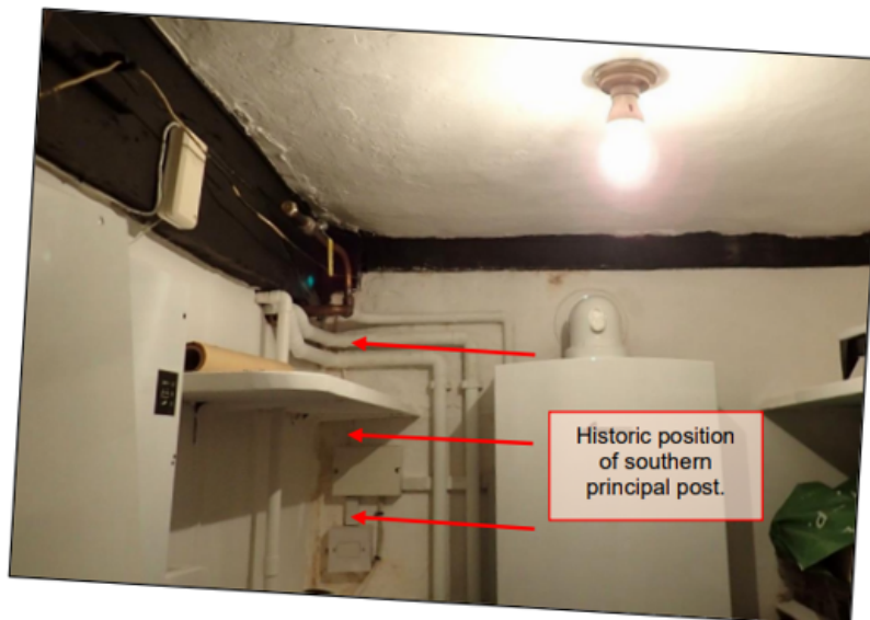
Figure 36. South-west corner of the Utility Room.
