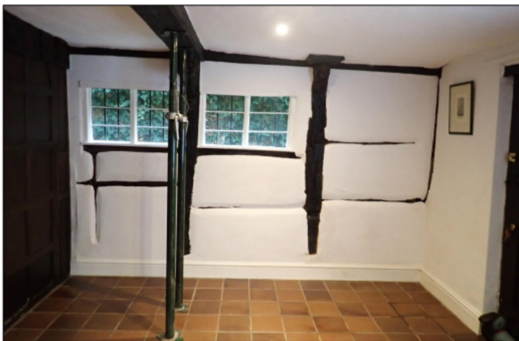
Figure 28. General view of the west wall from the Dining Room.
