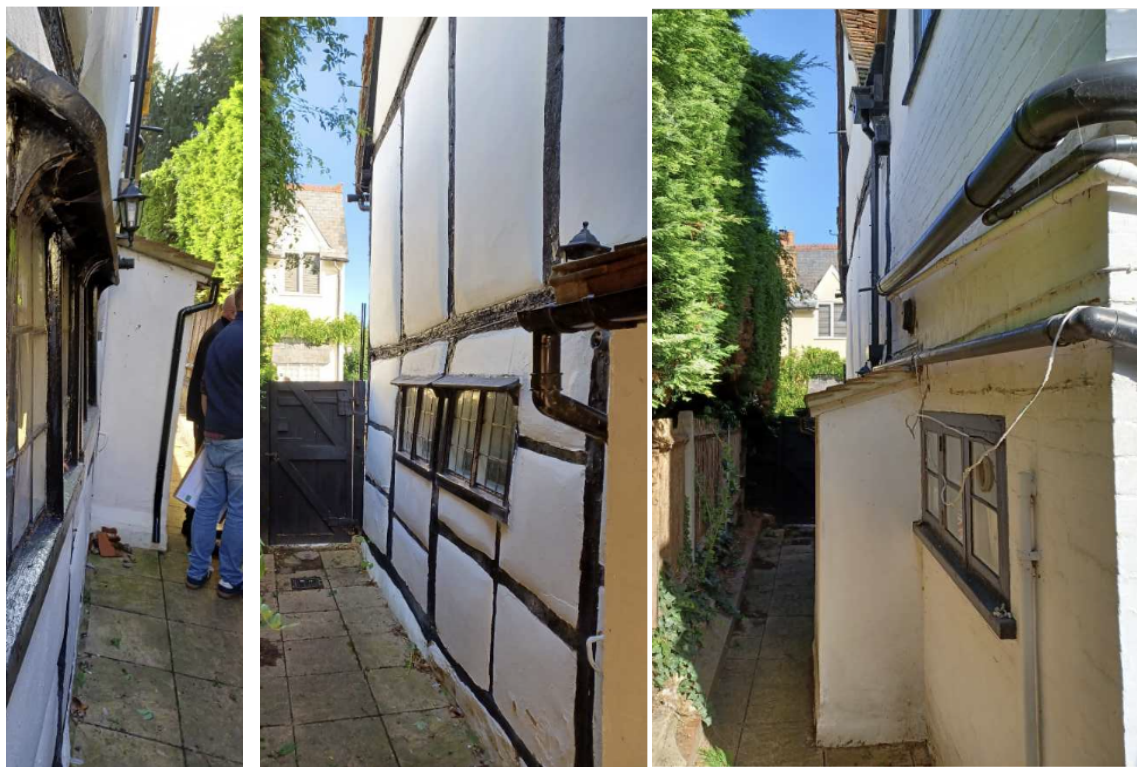
Western end gable, with far-right image being of the boiler extension.
