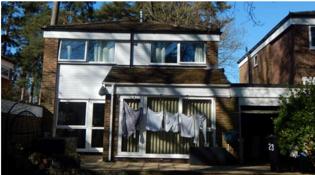
Image 2 – South facing elevation of the property
