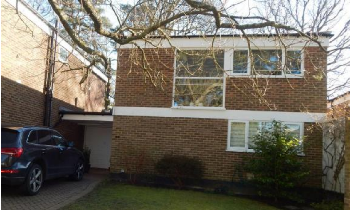
Image 1 – North facing elevation of the property
