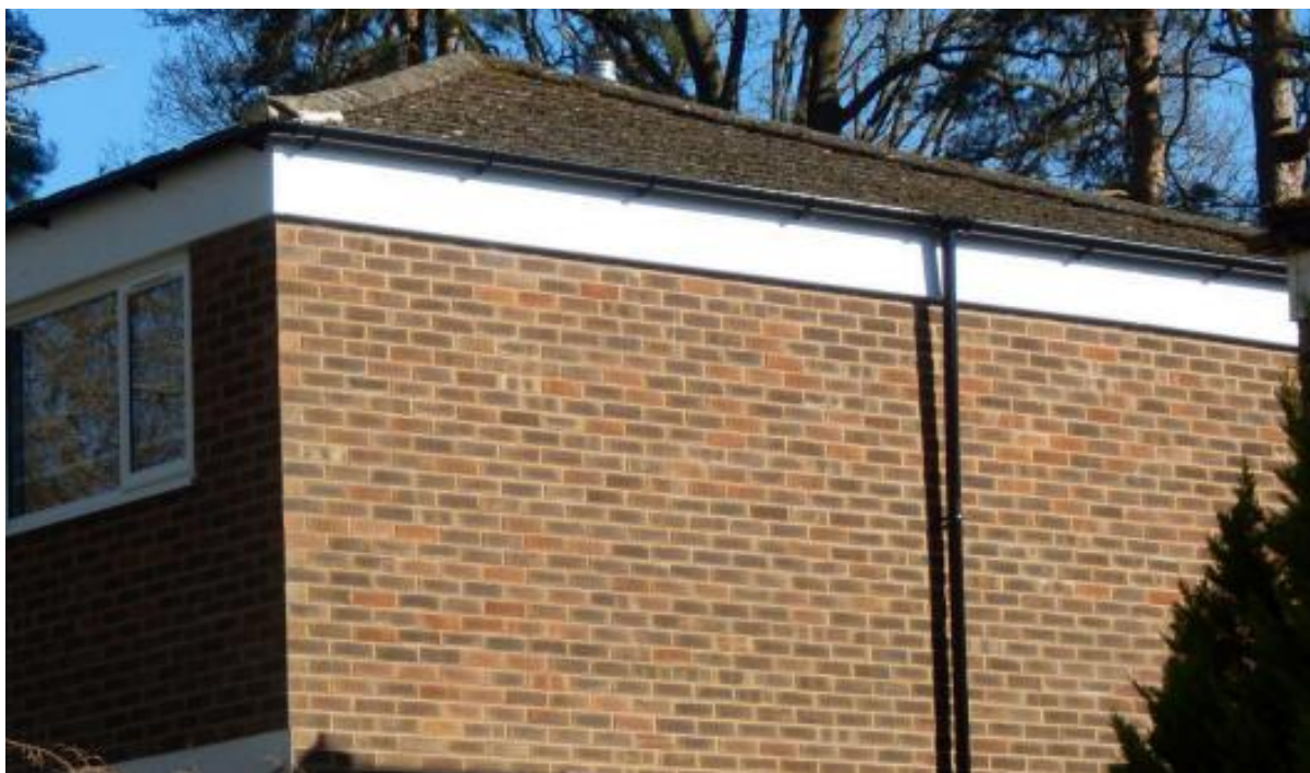
Image 4 – West facing elevation of the property
