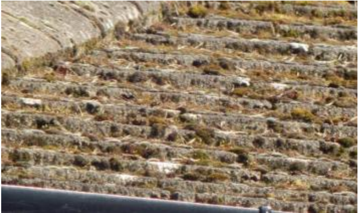
Image 5 – Close view of roof coverings to demonstrate condition
