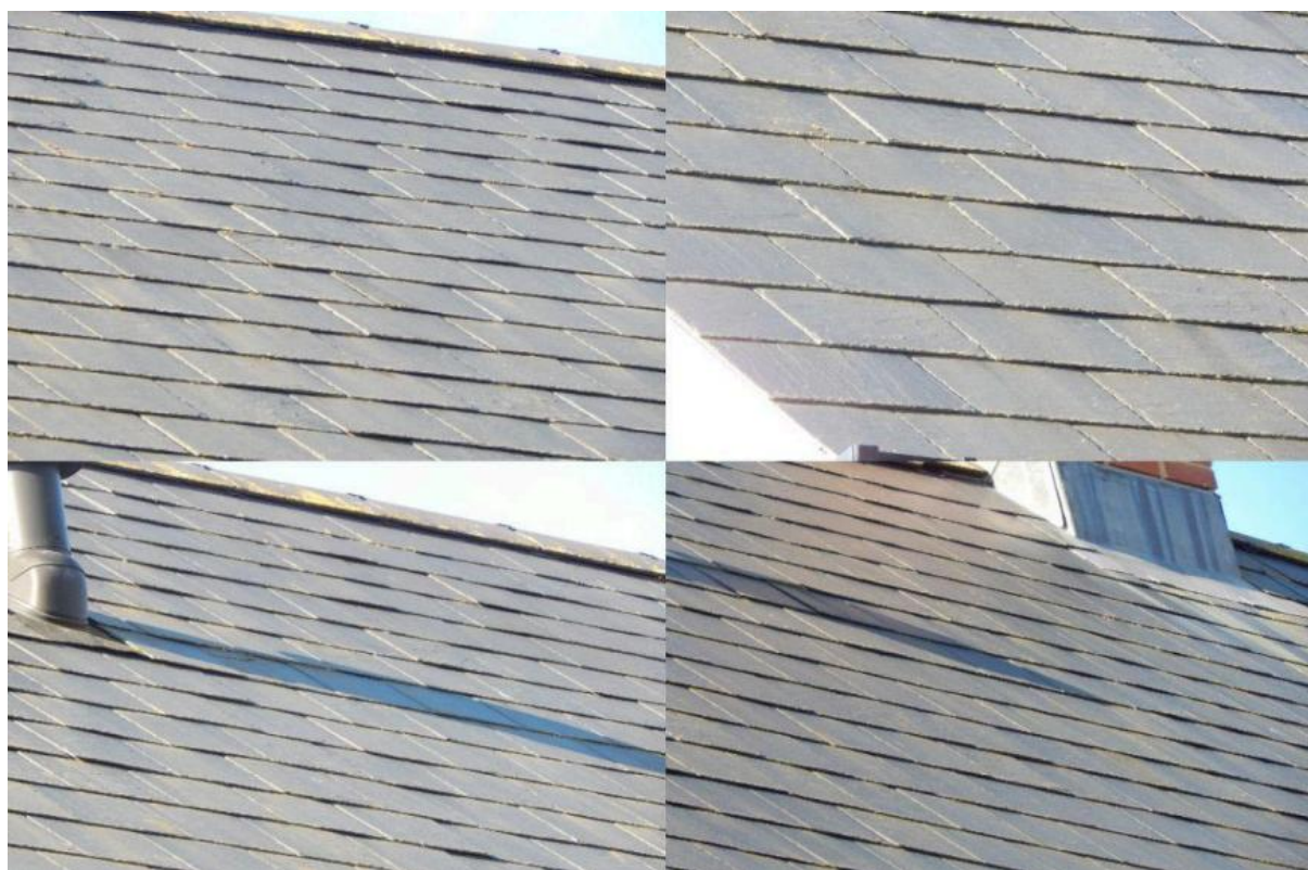
Image 4 – Close view of the South facing roof coverings
