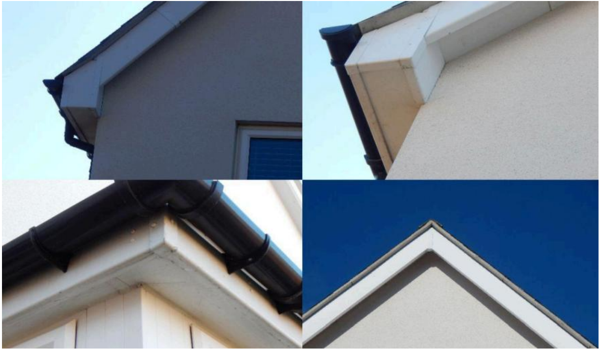
Image 7 – Close view of the eaves coverings
