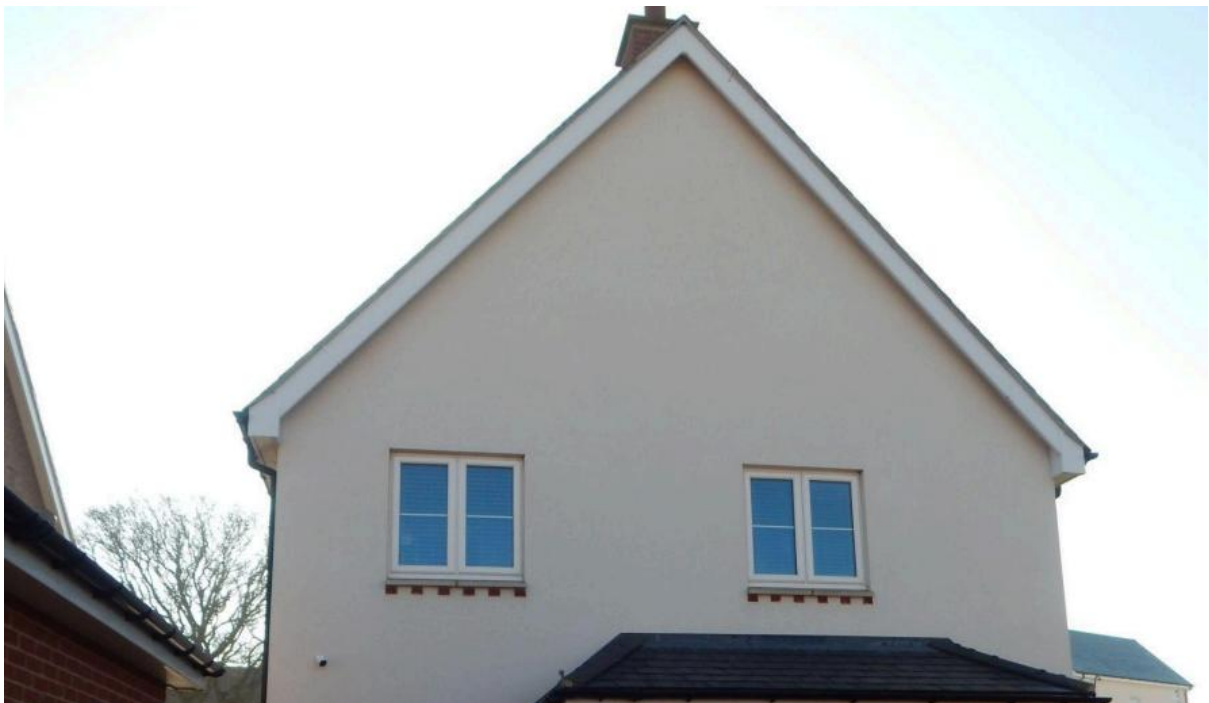
Image 6 – West facing elevation of the property
