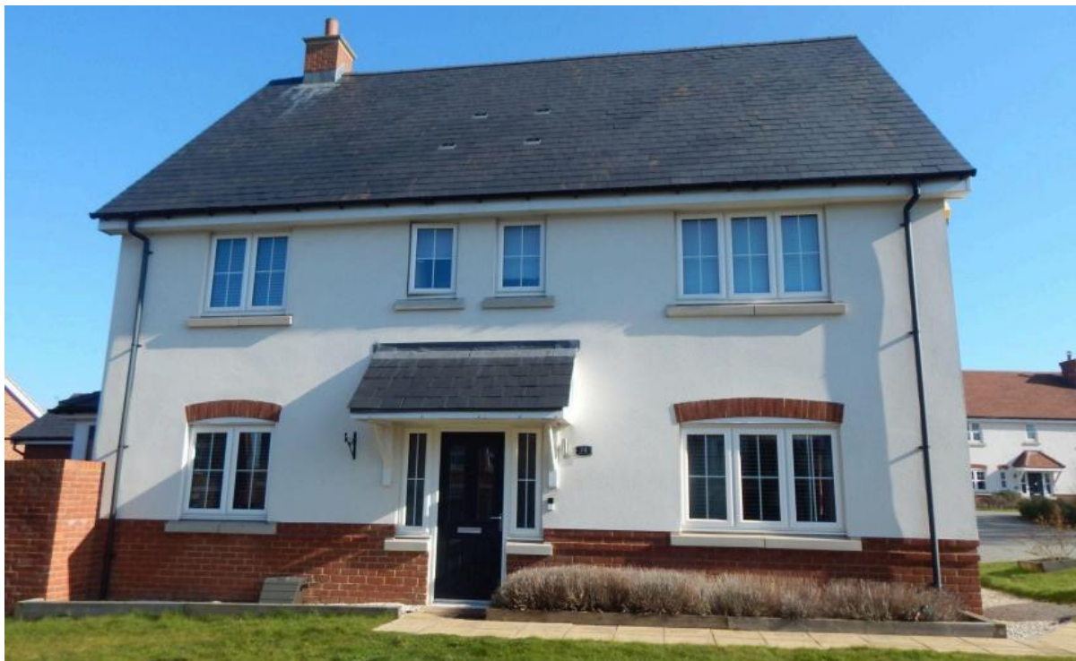
Image 1 – South facing elevation of the property
