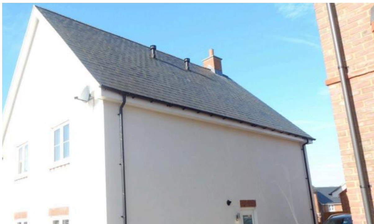
Image 3 – North facing elevation of the property
