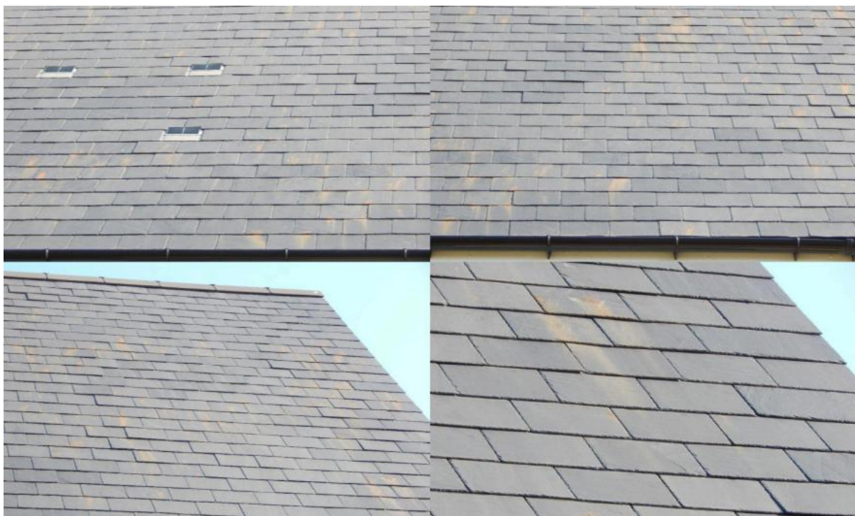
Image 2 – Close view of the South facing roof coverings
