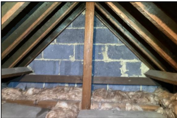
Photograph 5. Loft void showing fibreglass insulation.
