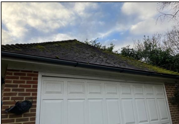
Photograph 7. Detached garage with flush roof tiles.
