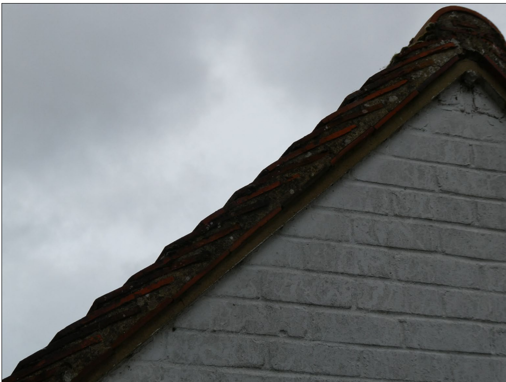
Figure 6. Example sealed verge. Bismillah House, Shinfield. 03.09.25
