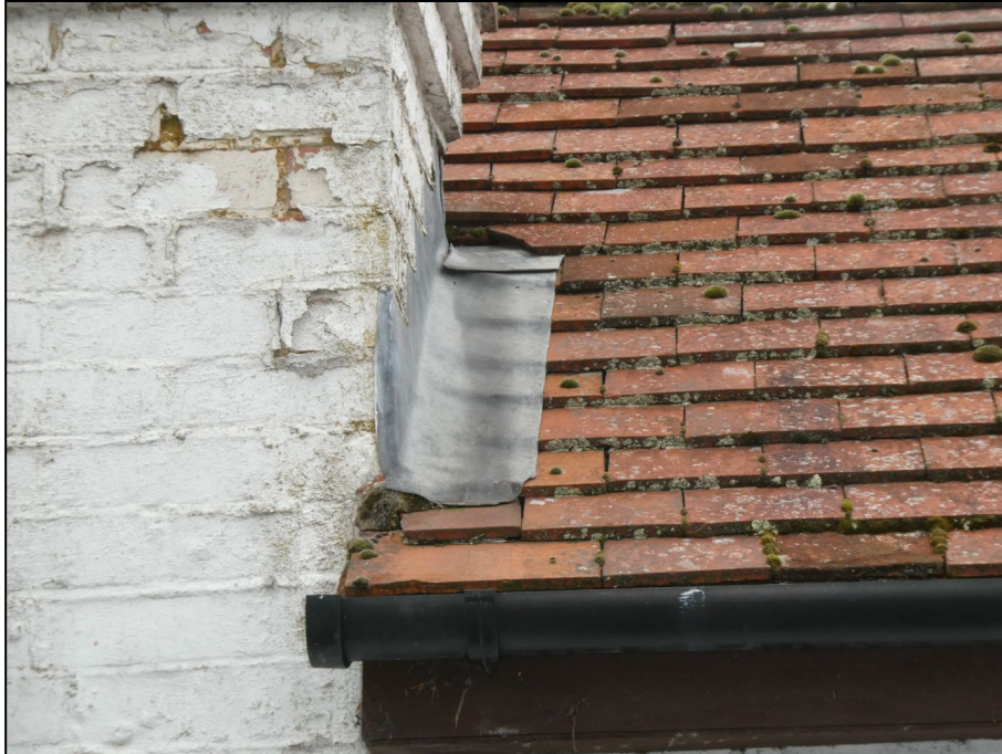
Figure 7. Example flush lead flashing. Bismillah House, Shinfield. 03.09.25
