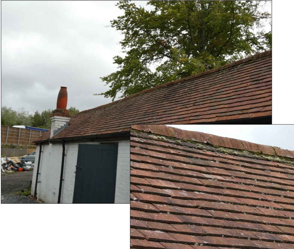
Figure 5. Example sealed ridge tiles. Bismillah House, Shinfield. 03.09.25
