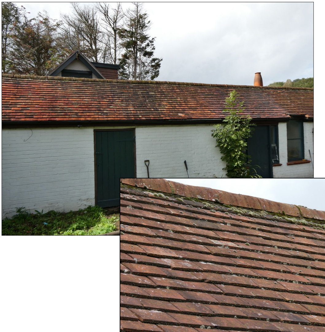
Figure 4. Roof over outbuilding at Bismillah House, Shinfield. 03.09.25
