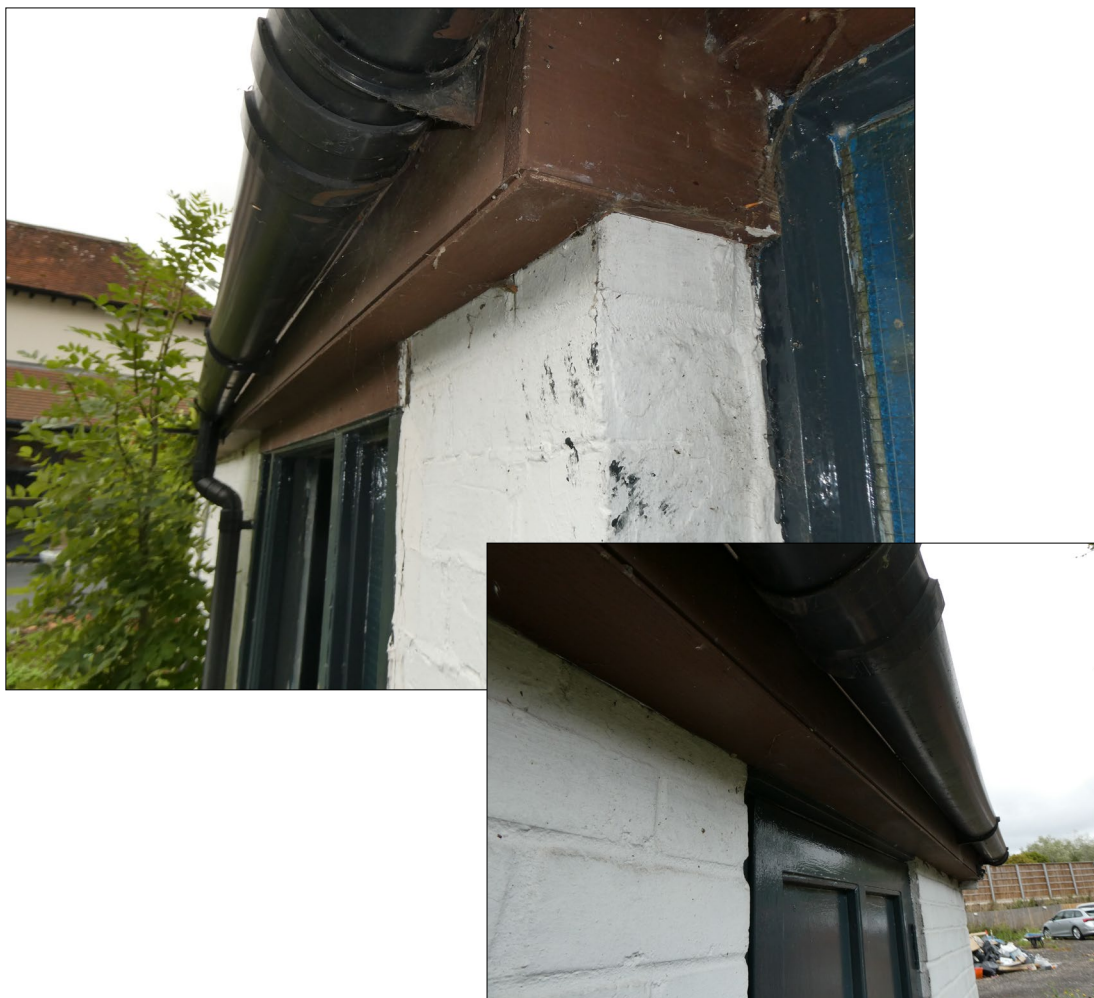
Figure 8. Example close fitted wooden soffits and fascias. Bismillah House, Shinfield. 03.09.25
