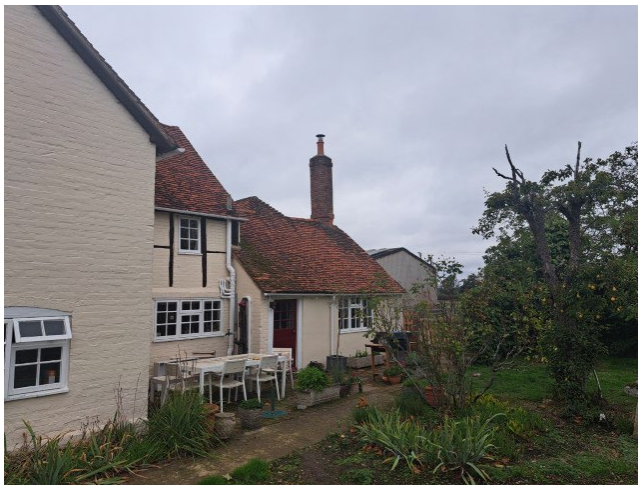
Photo 2-4 – View of the rear elevation of the farmhouse (east)
