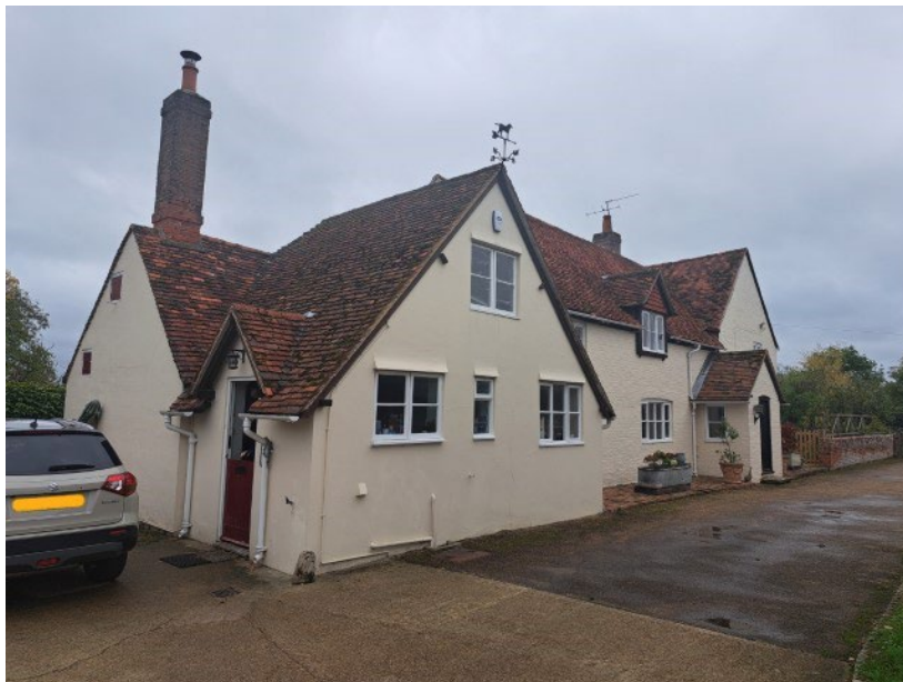
Photo 1 – View of front/side elevation of the farmhouse (northwest)
