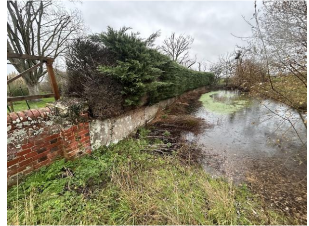
Photo 3: The pond to the south of the site, lined with a concrete wall.
