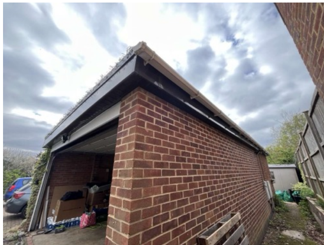
Photo 3: B2, northern elevation
