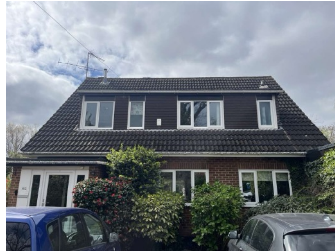
B1, main dwelling, northern elevation
