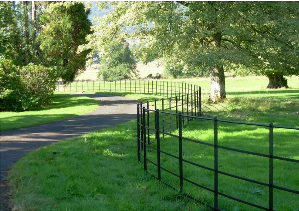
B02 (Q40/370) Estate rail Height: 1200mm Supplier: Britannia metalwork. Material: Wrought iron, weathered finish
