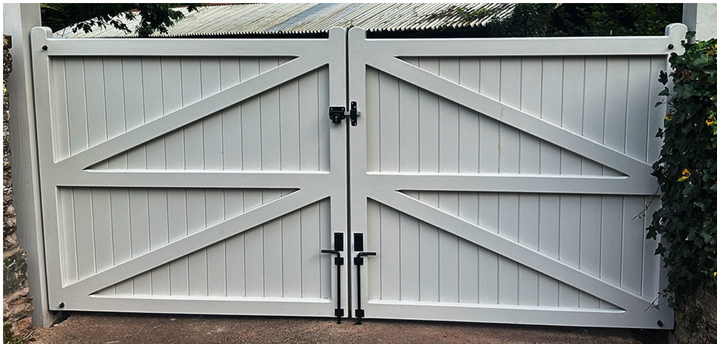
B10 (Q40/570) Timber gates Supplier: Suffolk Gates or similar painted grey
