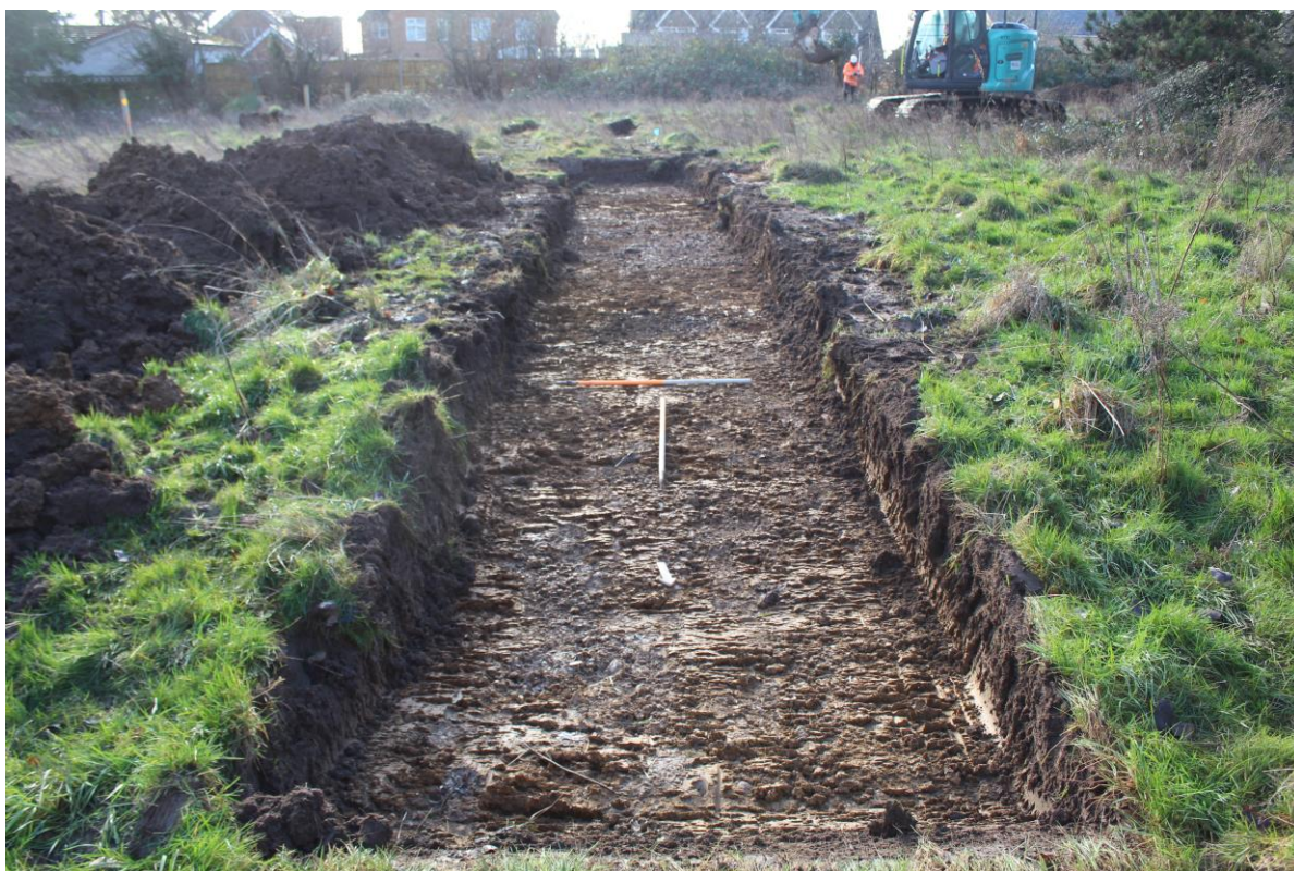
Plate 4: Trench 004, looking S (2 x 1m scale)
