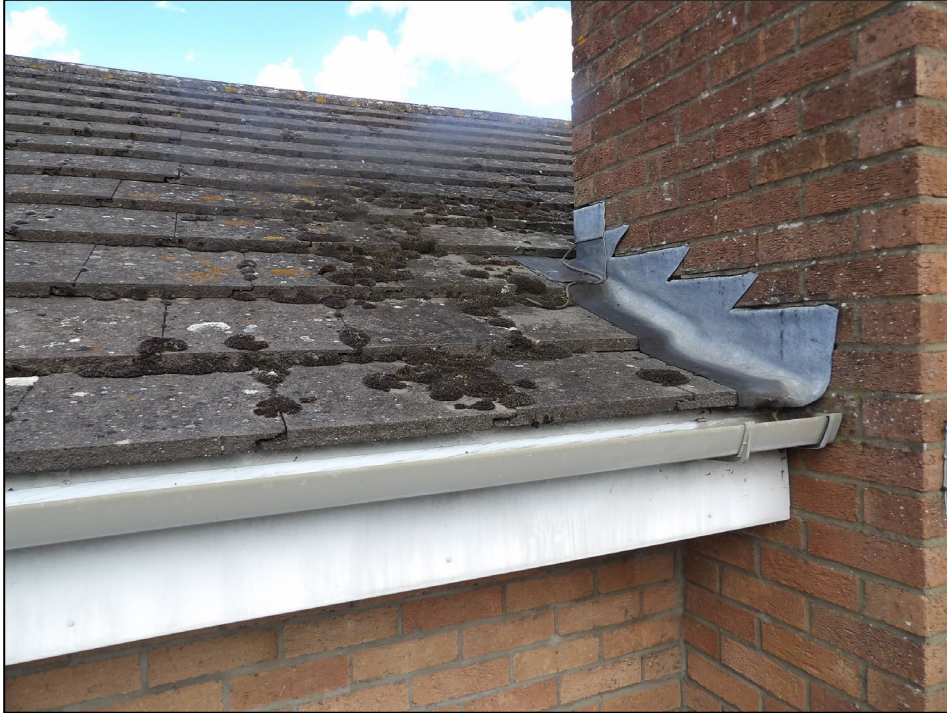
Figure 7. Example sealed lead flashing around chimney stack. 11 Retford Close, Woodley. 09.09.25
