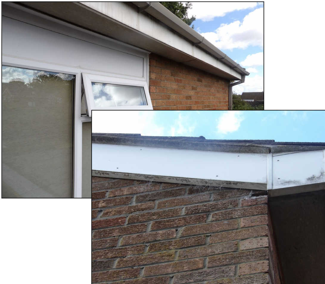
Figure 6. Example sealed uPVC soffits/fascias. 11 Retford Close, Woodley. 09.09.25
