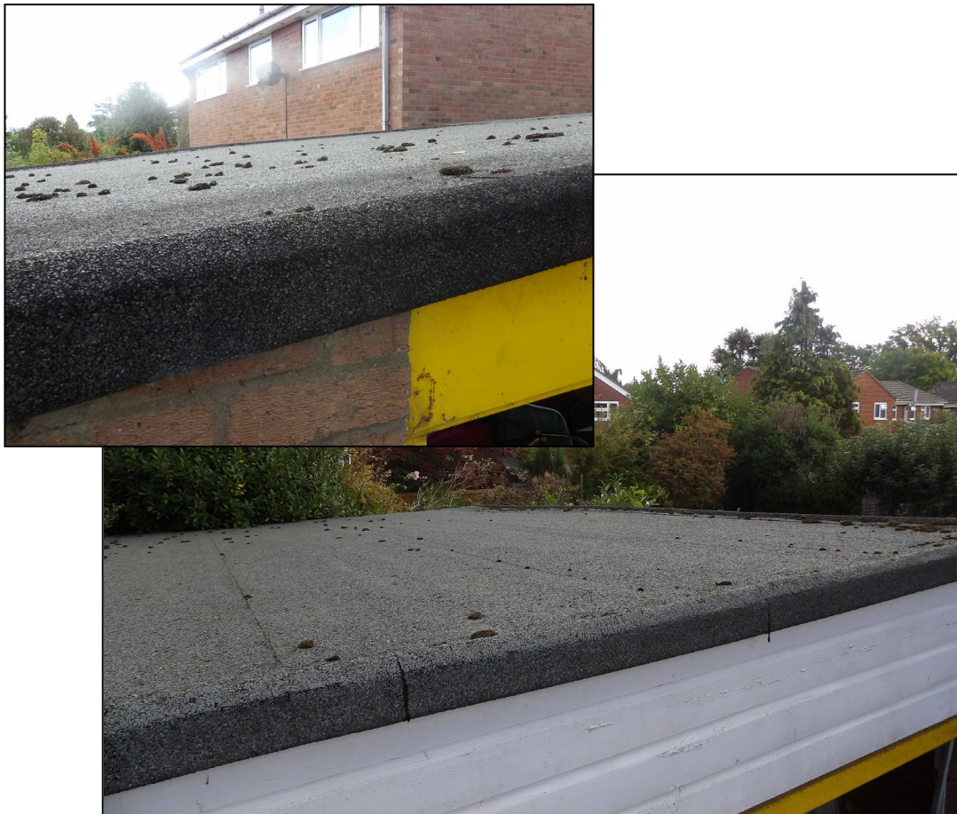
Figure 8. Example sealed bitumen felt on garage and sealed cladding. 11 Retford Close, Woodley. 09.09.25
