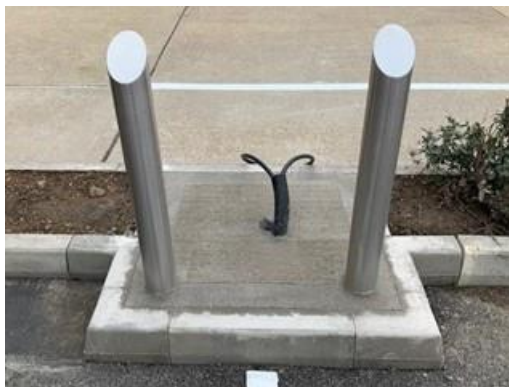
FIGURE 5: STAINLESS STEEL PROTECTION POSTS
