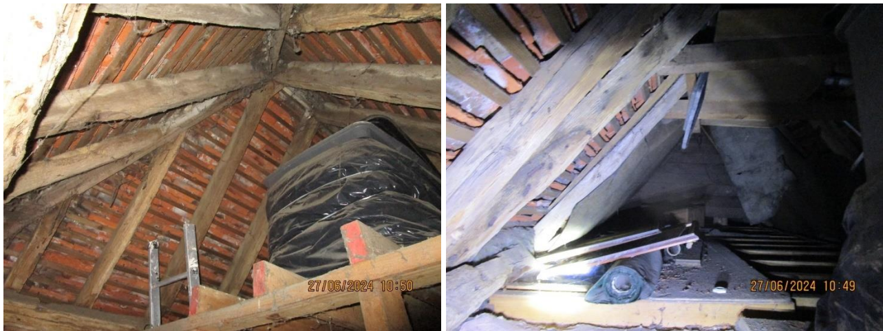
Photos 9 and 10 – Inside the main loft
