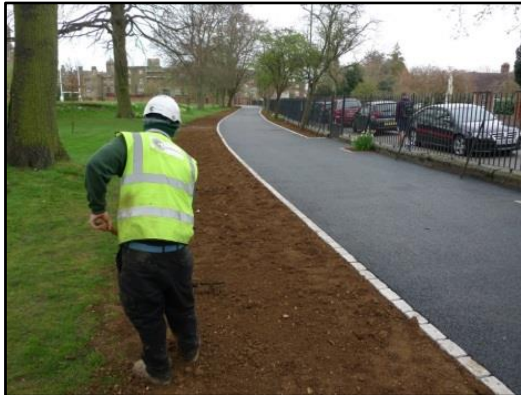
Fig 13 – All 'making good' topsoil will be BS3882 compliant and raked out by hand to no greater depth than 100mm.
