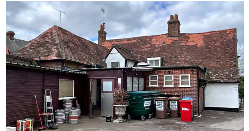
Fig 3.1 More modern rear extensions with flat roofs
