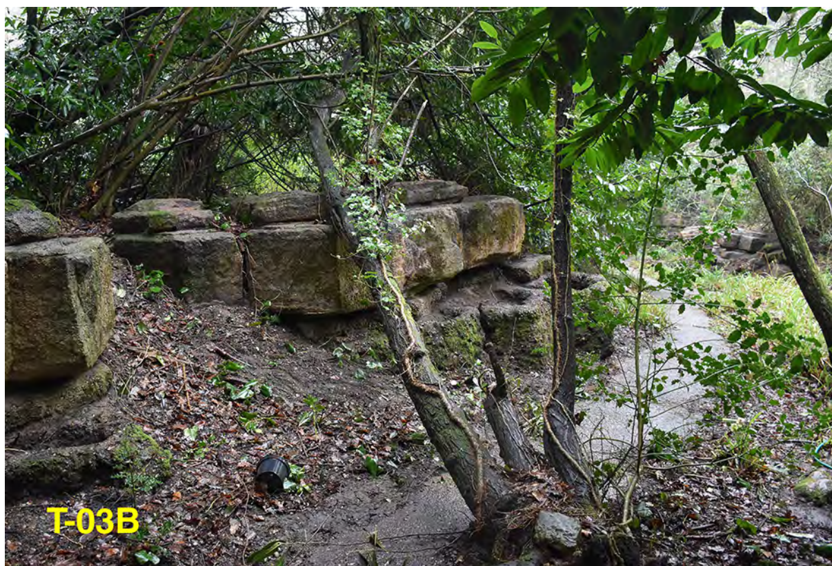
06: TREE T-03 FALLEN ACROSS PATH & NOW RESTING ON PULHAMITE
