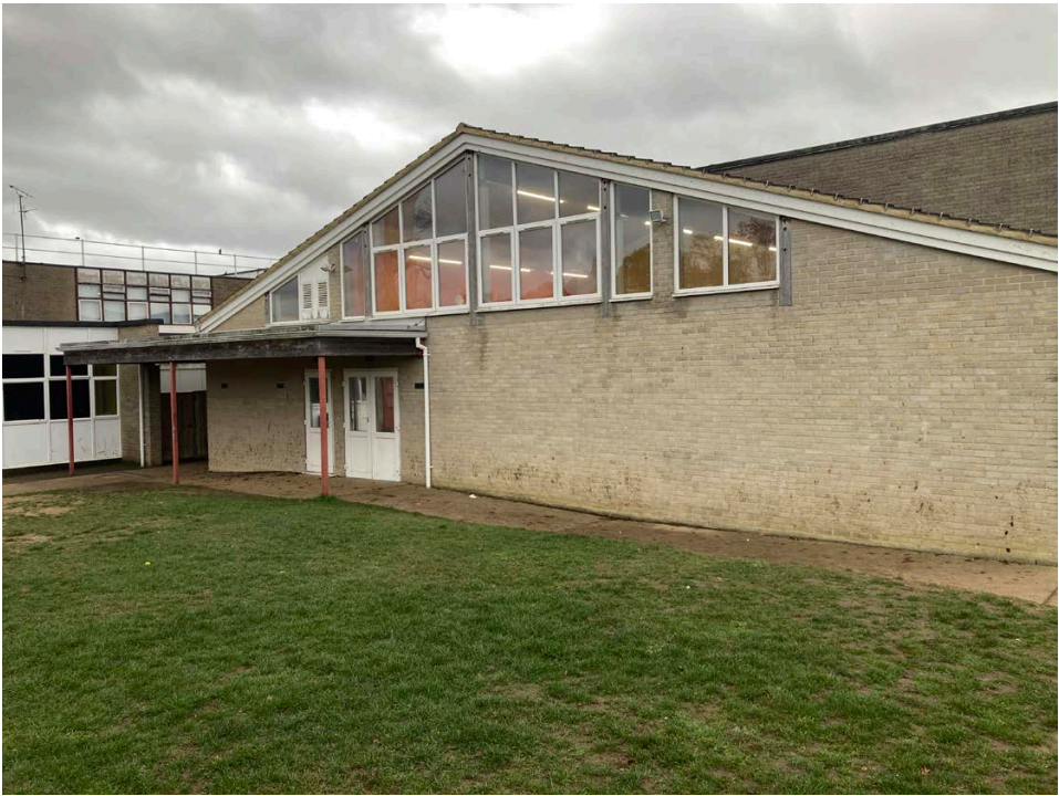
North west face of gym
