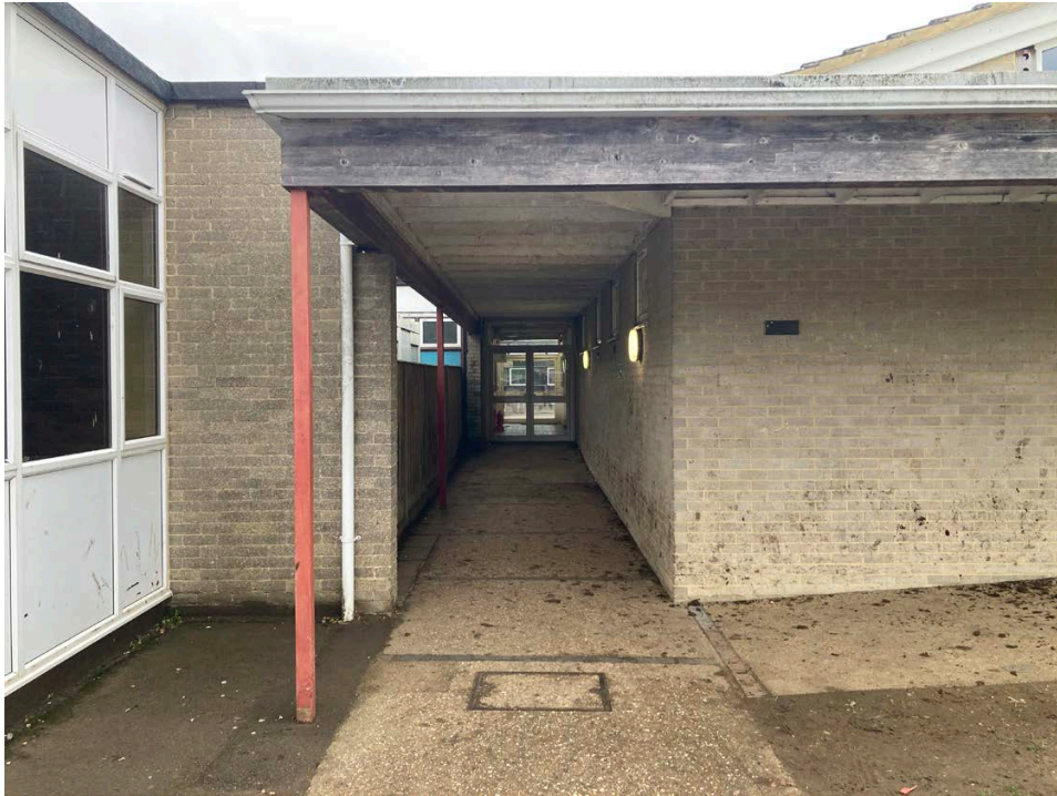
Circulation route to rear of gym
