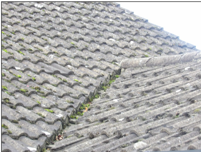
Figure 5. Example sealed ridge tiles and valleys on front elevation. 372 Reading Road, Winnersh. 04.11.25
