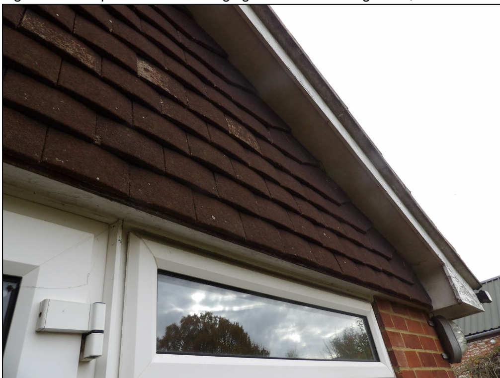
Figure 9. Example close fitted hanging tiles. 372 Reading Road, Winnersh. 04.11.25
