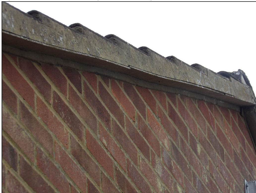
Figure 7. Example sealed verges. 372 Reading Road, Winnersh. 04.11.25
