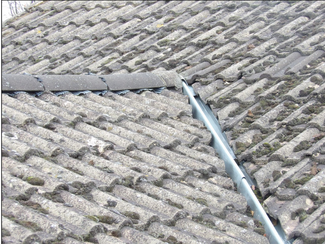
Figure 6. Example dry ridge and valley on rear elevation. 372 Reading Road, Winnersh. 04.11.25
