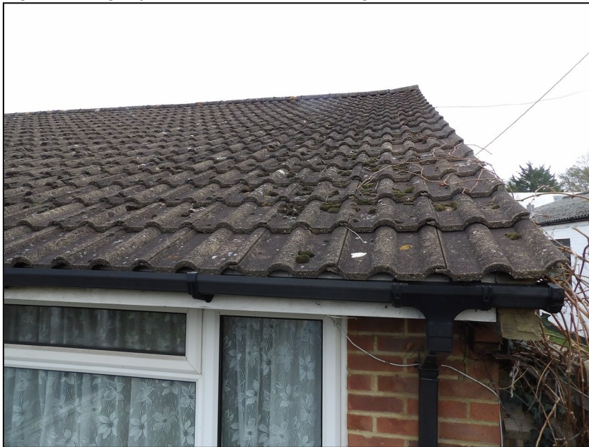
Figure 4. Tightly fitted roof. 372 Reading Road, Winnersh. 04.11.25
