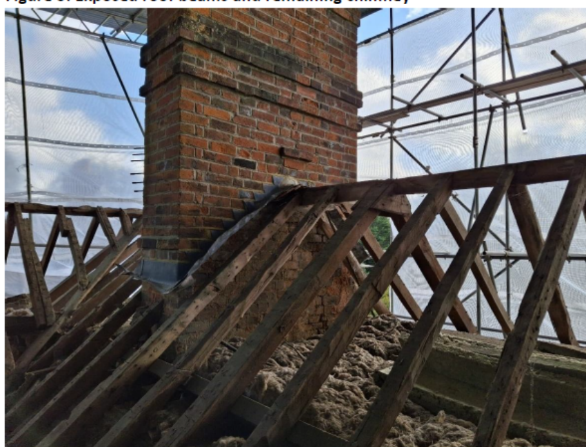
Figure 3: Exposed roof beams and remaining chimney
