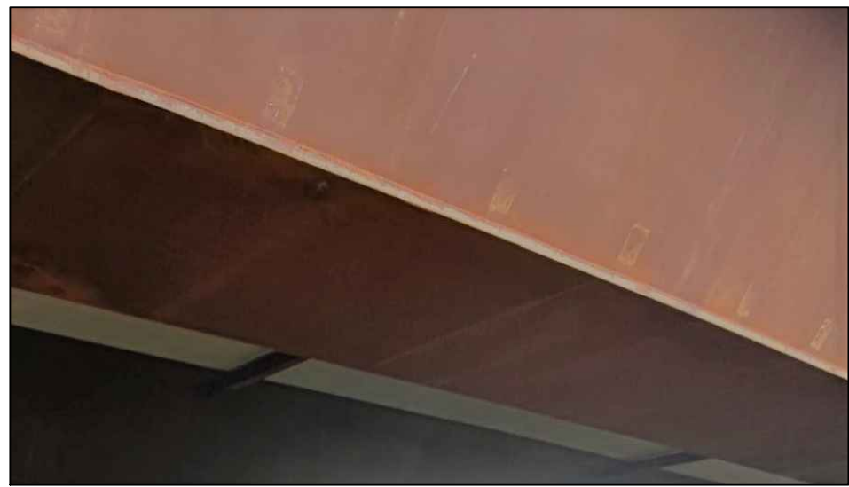
DETAIL 3 - WEATHERING STEEL BOX GIRDER (SEE NOTE 4)
