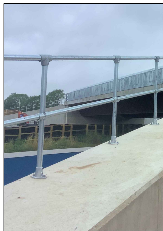
DETAIL 10 - GUARD RAIL ON WINGWALLS (SEE NOTE 4)
