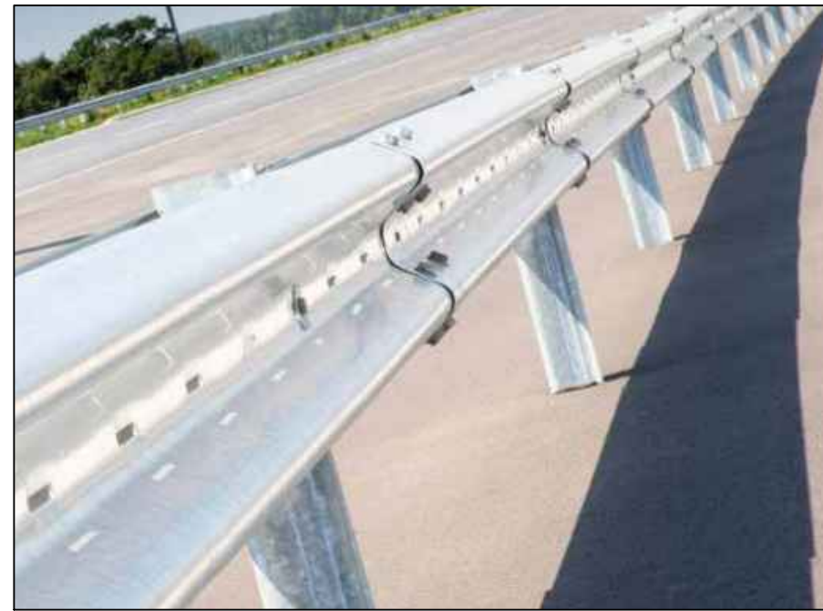
DETAIL 2 - SAFETY BARRIER
