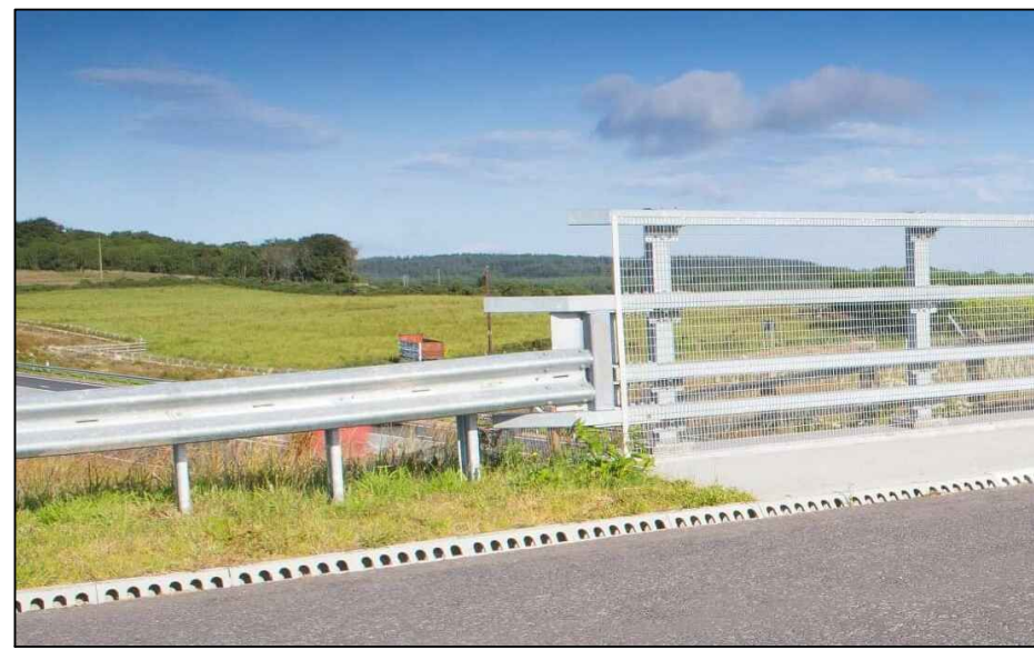
DETAIL 1 - PARAPET TO SAFETY BARRIER TRANSITION
