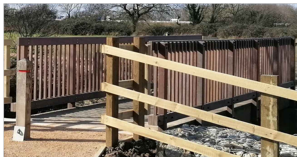
DETAIL 11 - EKKI TIMBER BOARDWALK AND FOOTBRIDGE (SEE NOTE 6)
