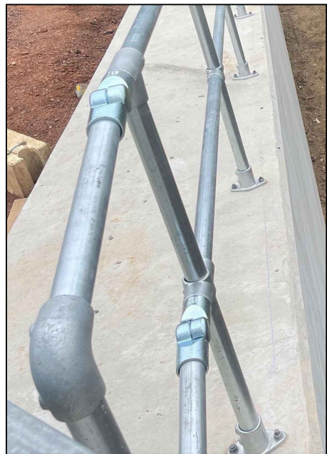
DETAIL 9 - GUARD RAIL ON WINGWALLS (SEE NOTE 4)
