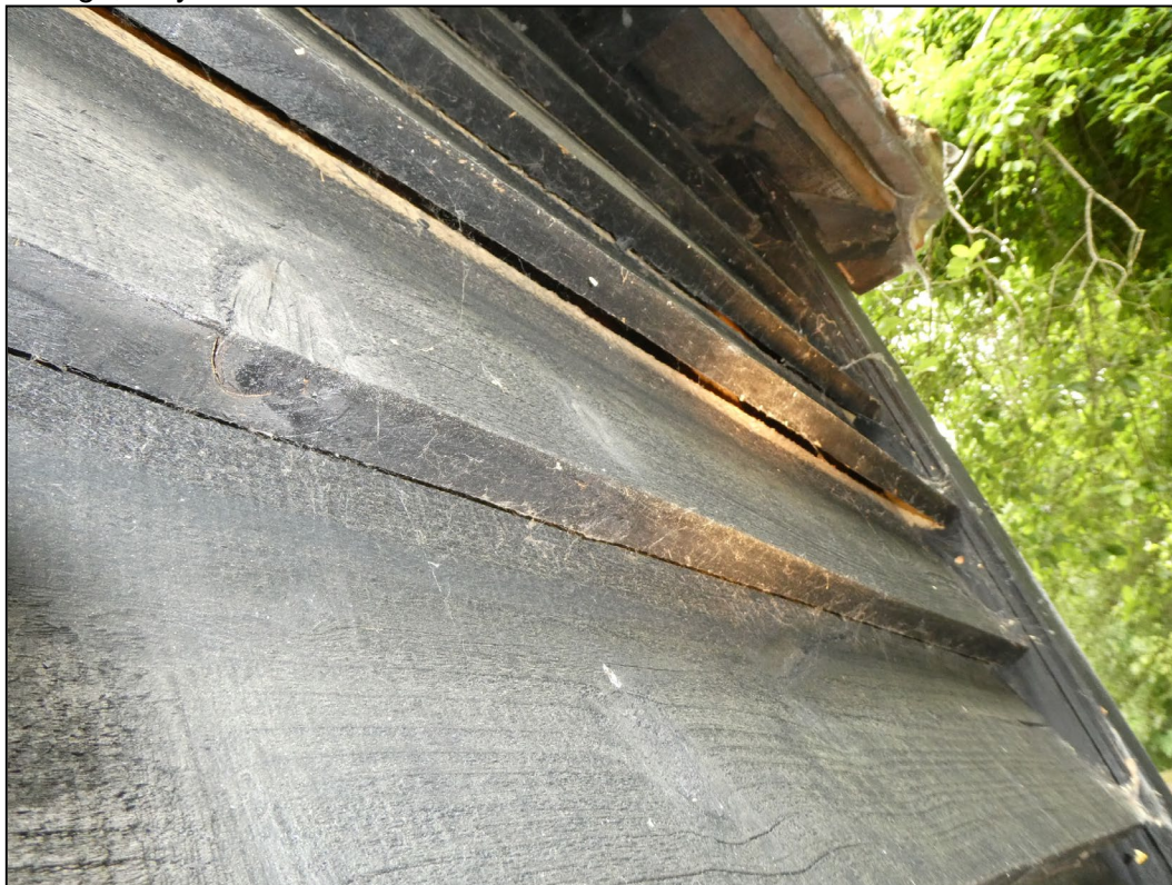
Figure 7. Example warped timber cladding. Granary building at Stanlake Farm Cottage, Twyford. 03.06.25
