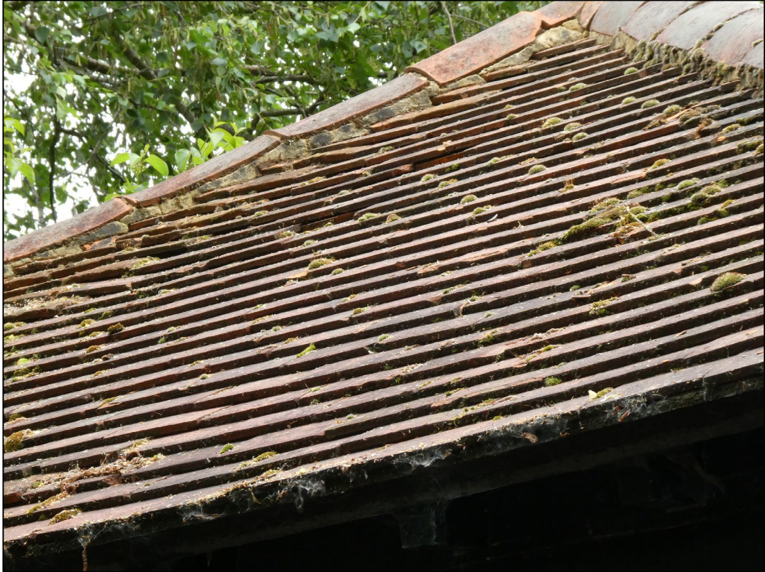
Figure 5. Example raised/broken roof tiles. Granary building at Stanlake Farm Cottage, Twyford. 03.06.25
