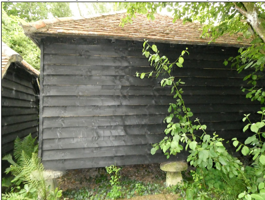
Figure 4. Rear view of granary building at Stanlake Farm Cottage, Twyford. 03.06.25
