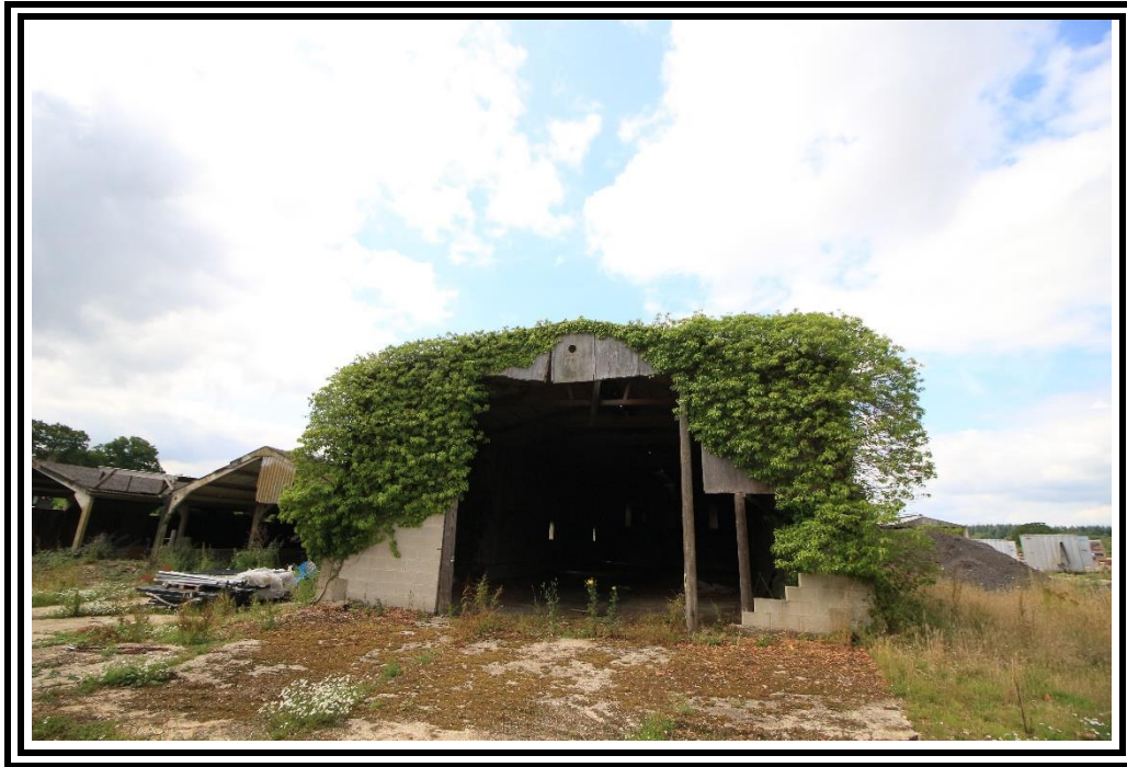
Photo 11: Building B: Rear elevation
