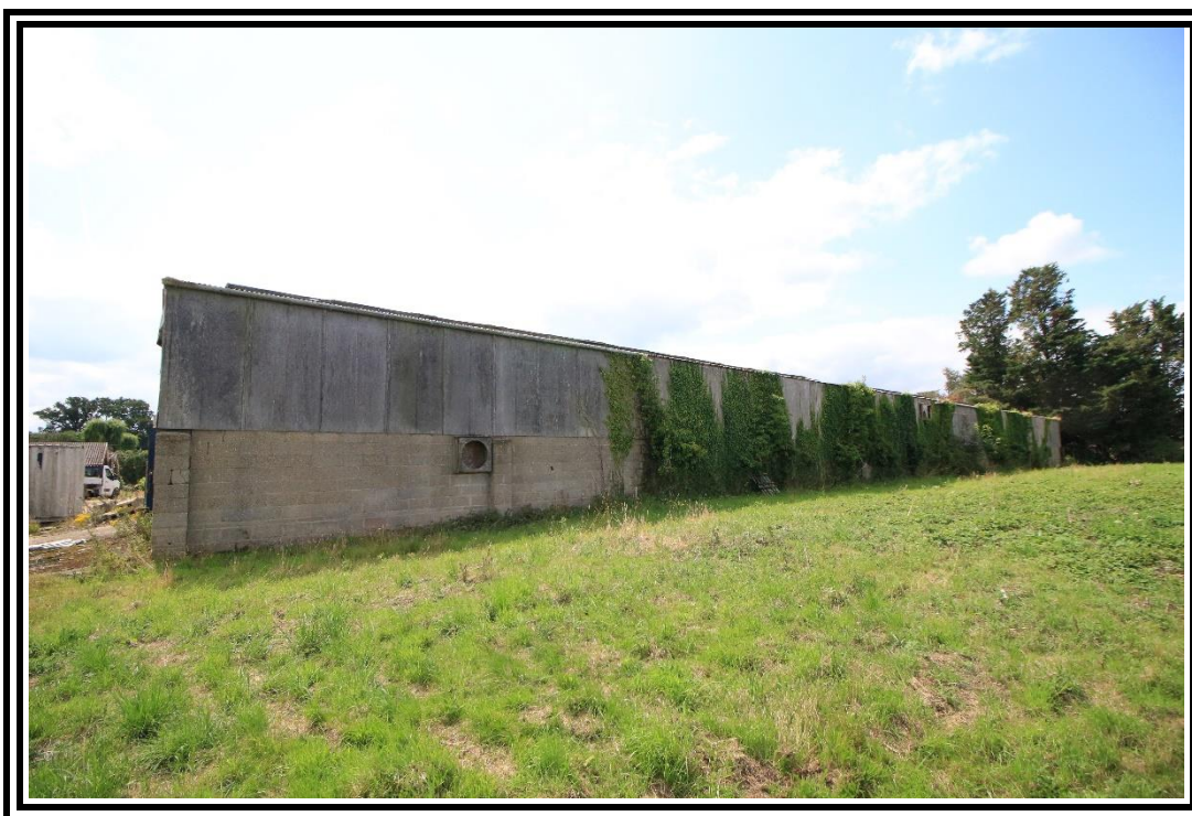
Photo 4: Building A: North side elevation
