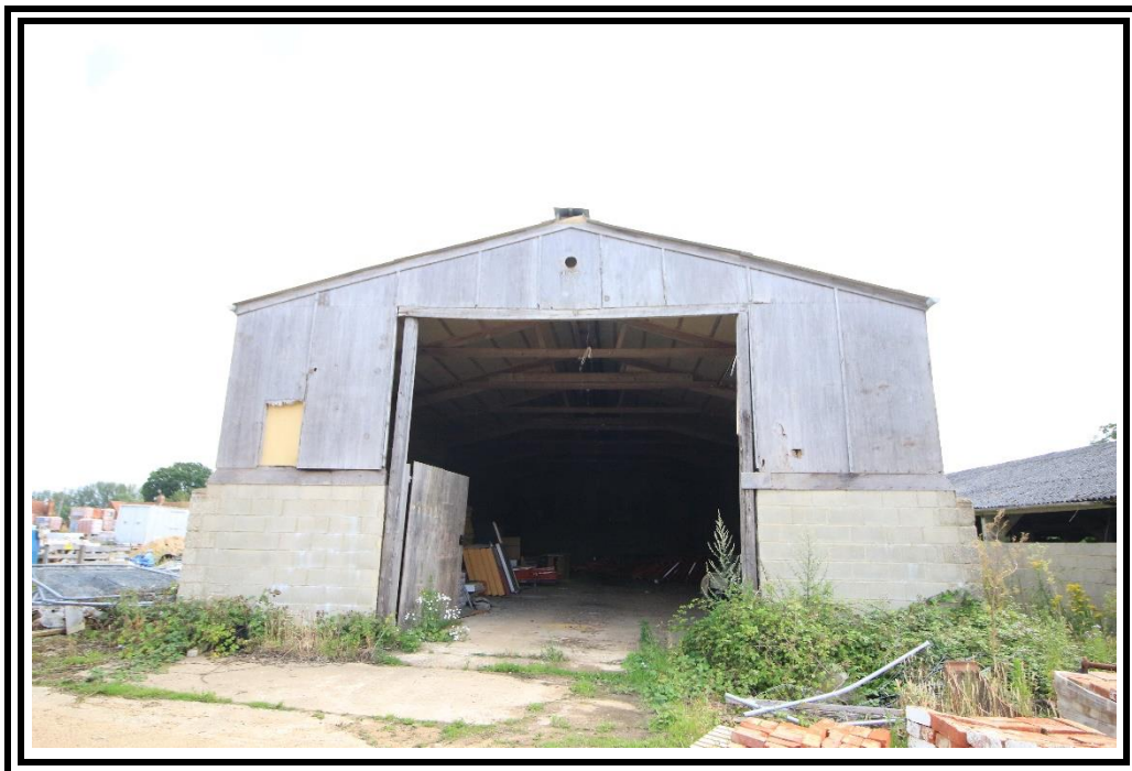
Photo 10: Building B Front elevation
