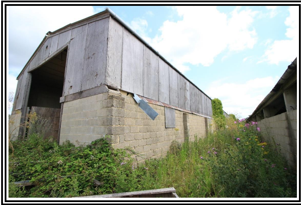
Photo 9: Building B South elevation
