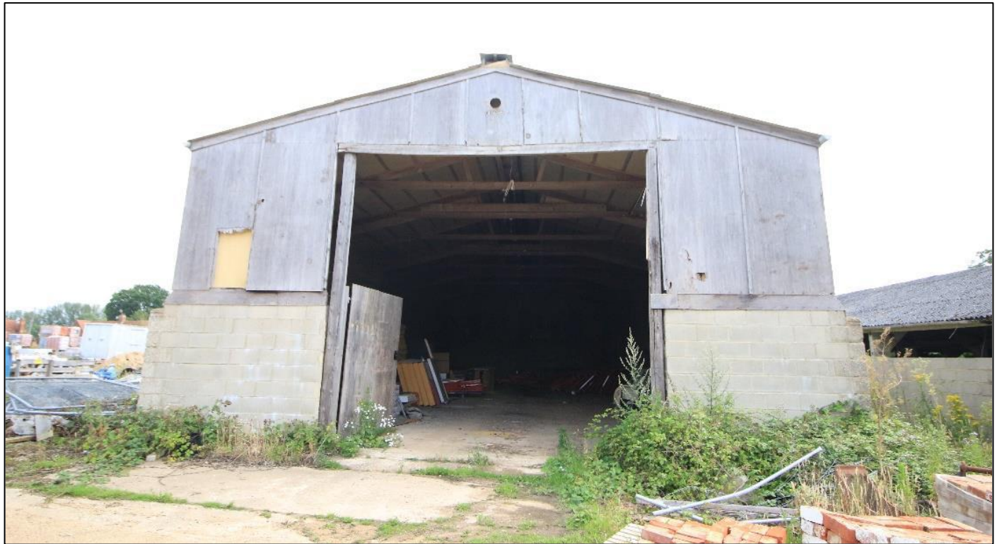
Figure 2: Barn B, west elevation from structural survey July 2024
