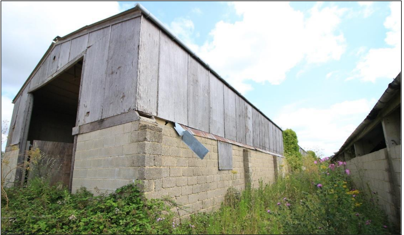
Figure 3: Barn B, south and west elevations from structural survey July 2024
