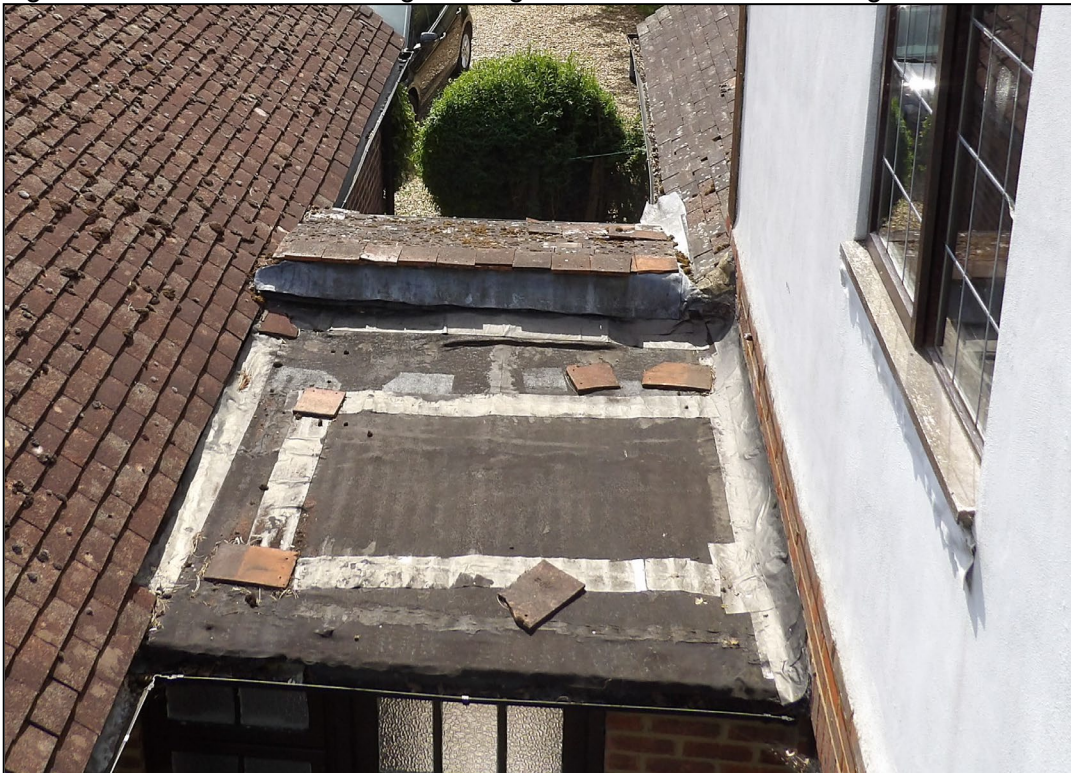
Figure 10. Roof of link attaching building. 6 Old Bath Road, Sonning. 20.05.25
