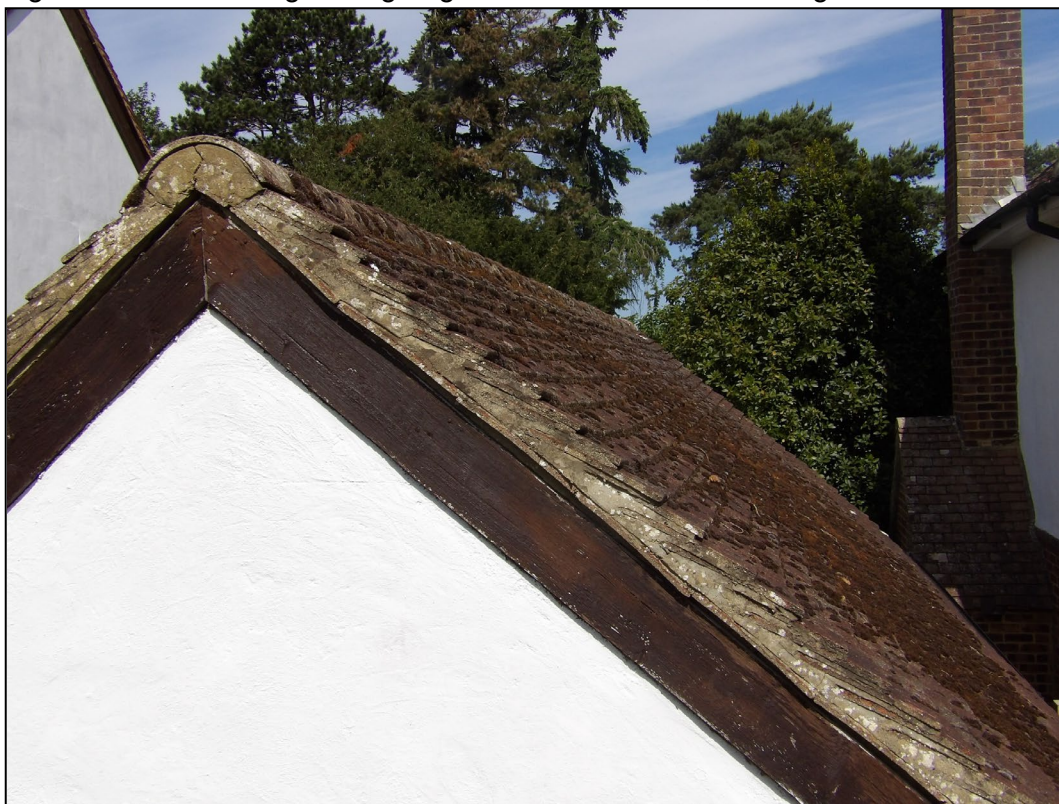
Figure 13. Sealed verges on garage. 6 Old Bath Road, Sonning. 20.05.25
