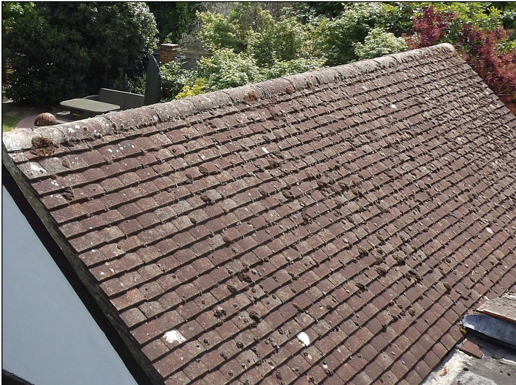
Figure 12. Well fitted roof and ridge tiles on garage. 6 Old Bath Road, Sonning. 20.05.25
