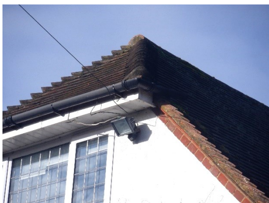
9. Verge mortar tight to the brickwork at the front of the house.
