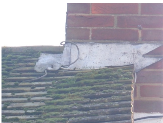
7. Lead flashing tight around the chimney.
