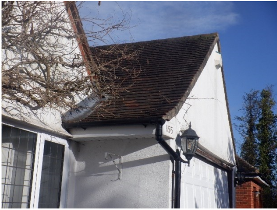
13. Roof and ridge tiles tight in place and tightly fitted, with a few gaps along the verge of the garage.
