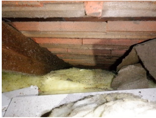
20. Eaves filled with fibreglass.
