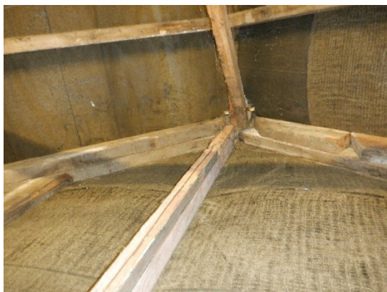
25. Cobwebbed ridge of the garage.
