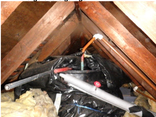
15. Internal view of the roof space viewing north.
