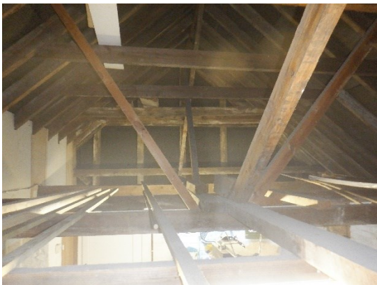
23. Interior of the garage.
