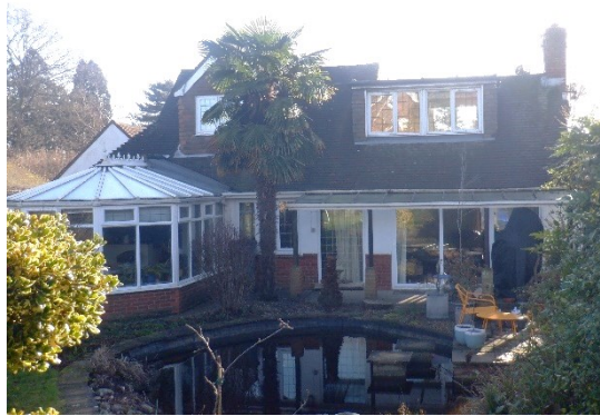
2. Rear of the house viewed from the north.
