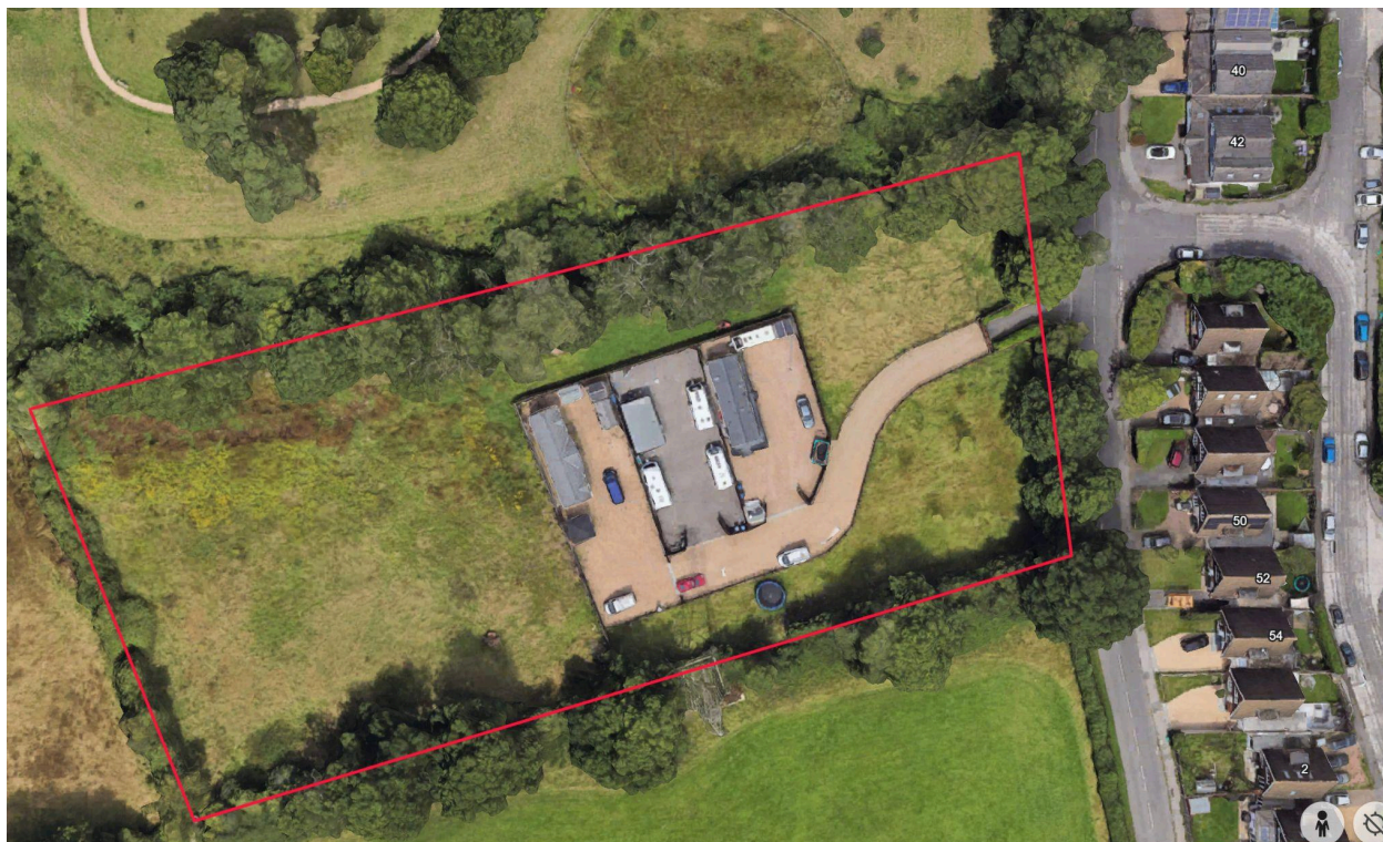
Surveyed area within red line boundary.
