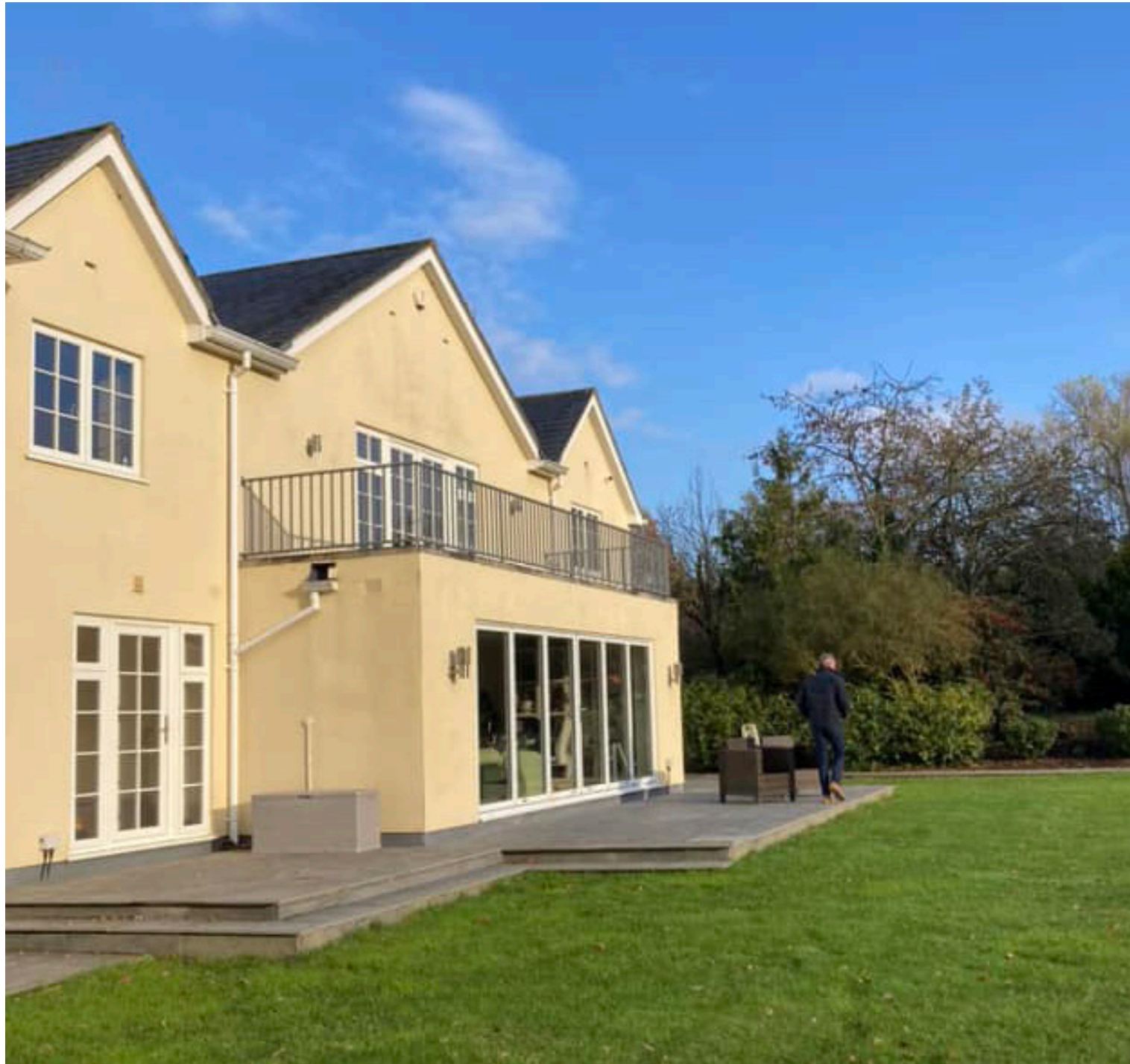
The south side of the existing house
