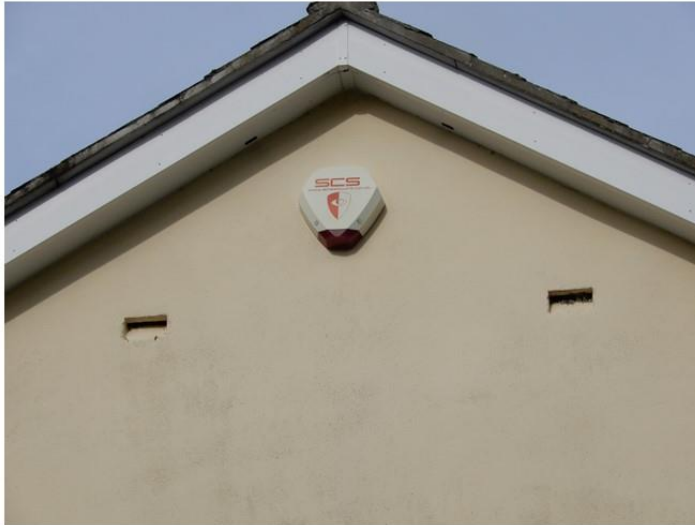
Photograph 7 — Integrated bat boxes present within the main house. Likely a result of the recorded EPSL for roosting brown long-eared, common pipistrelle, and soprano pipistrelle bats on site.
