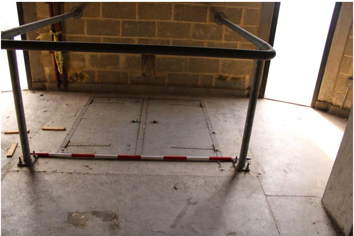
Photograph 49. Illustrative View of Missing Lift Shaft
