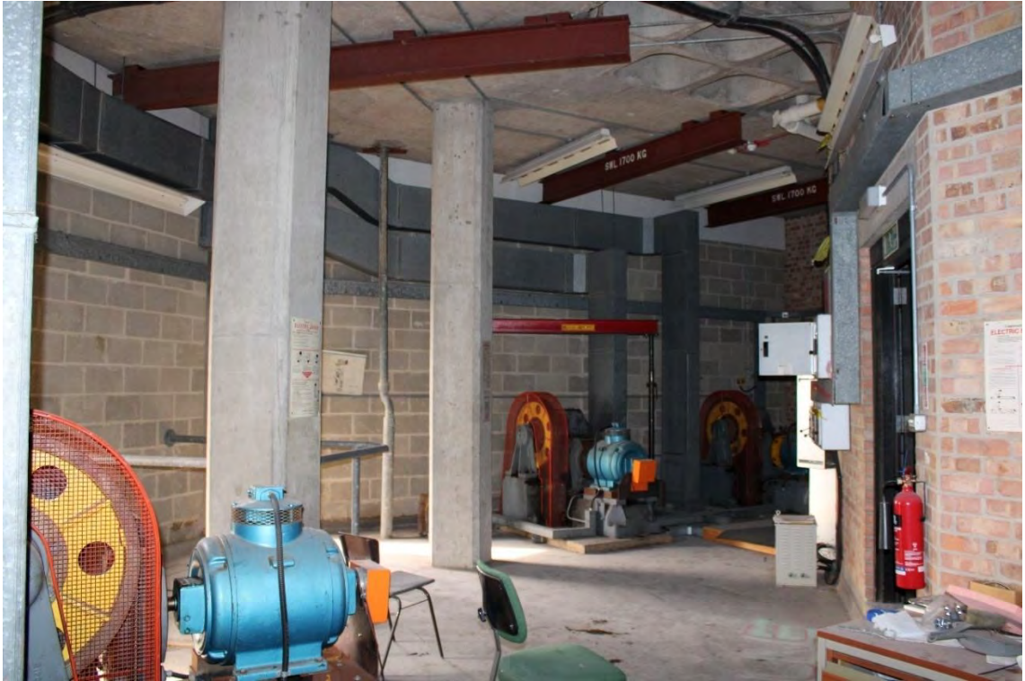
Photograph 48. Illustrative View of Lift Motor Room
