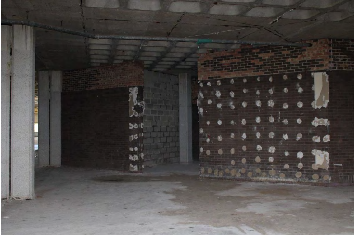
Photograph 40. Illustrative View of Dot and Dab Plaster
