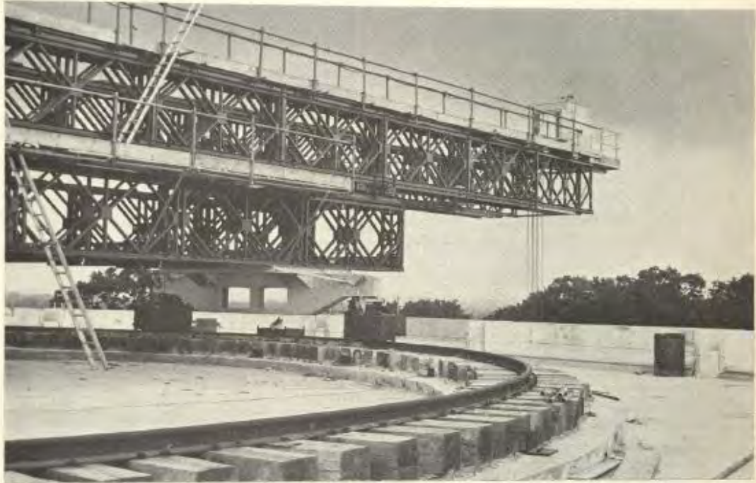
The Bailey bridge panel placer and concrete ring beam used for lifting the cladding panels.
