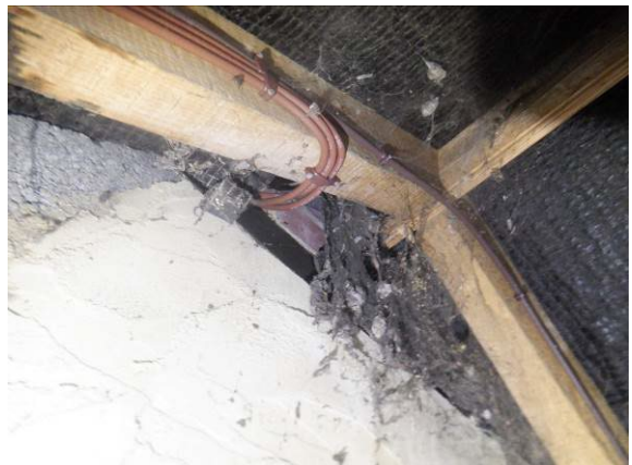
Photograph 20. Slope at apex of western gable (roof void).
