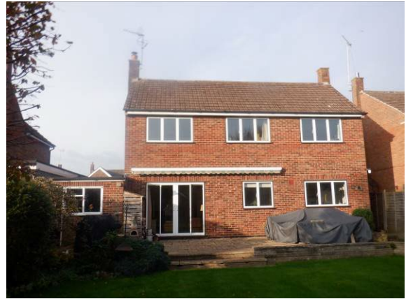
Photograph 2. Rear of property viewed from south.
