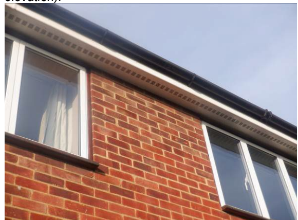
Photograph 6. Tight uPVC soffits (rear elevation).
