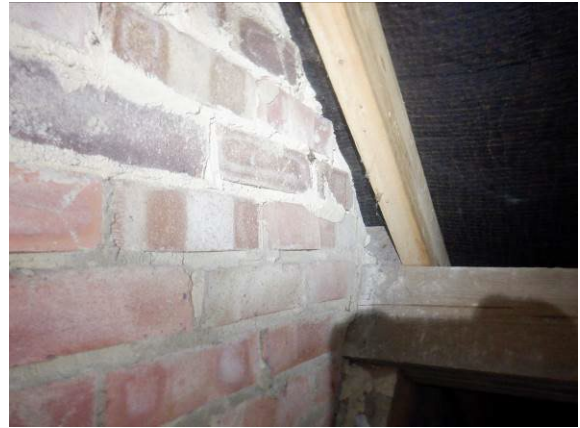
Photograph 18. Front northern gable end (roof void).
