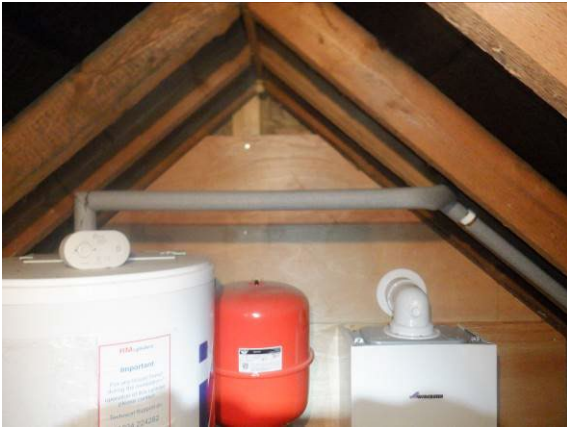
Photograph 17. Eastern gable end (roof void).
