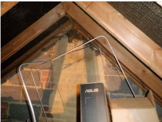
Photograph 19. Western gable end (roof void).
