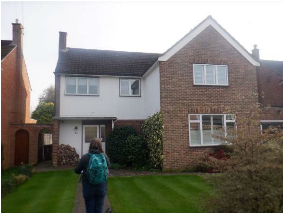
Photograph 1. Front of property viewed from north.
