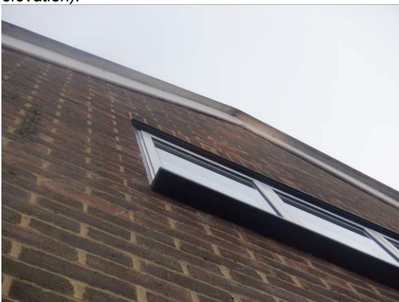
Photograph 5. Flush uPVC barge boards on front gable (front elevation).
