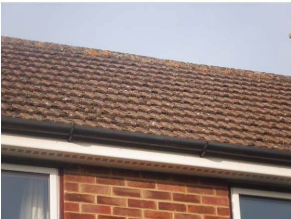
Photograph 3. Interlocking roof tiles (rear elevation).
