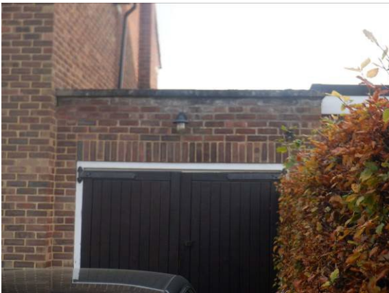
Photograph 11. Front of garage viewed from north.
