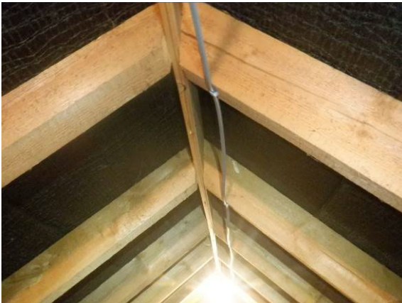
Photograph 15. Intact bitumen roofing felt (roof void).
