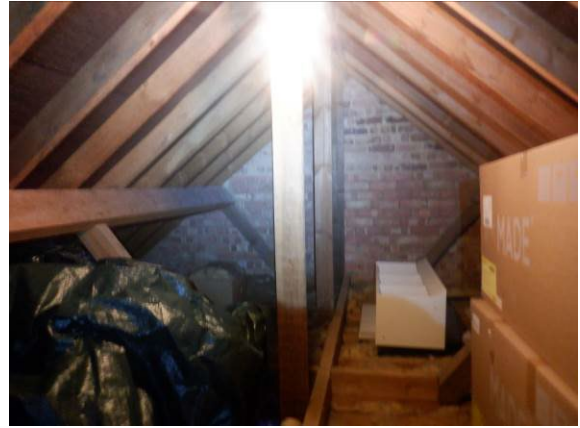
Photograph 14. Front gable extension (roof void).
