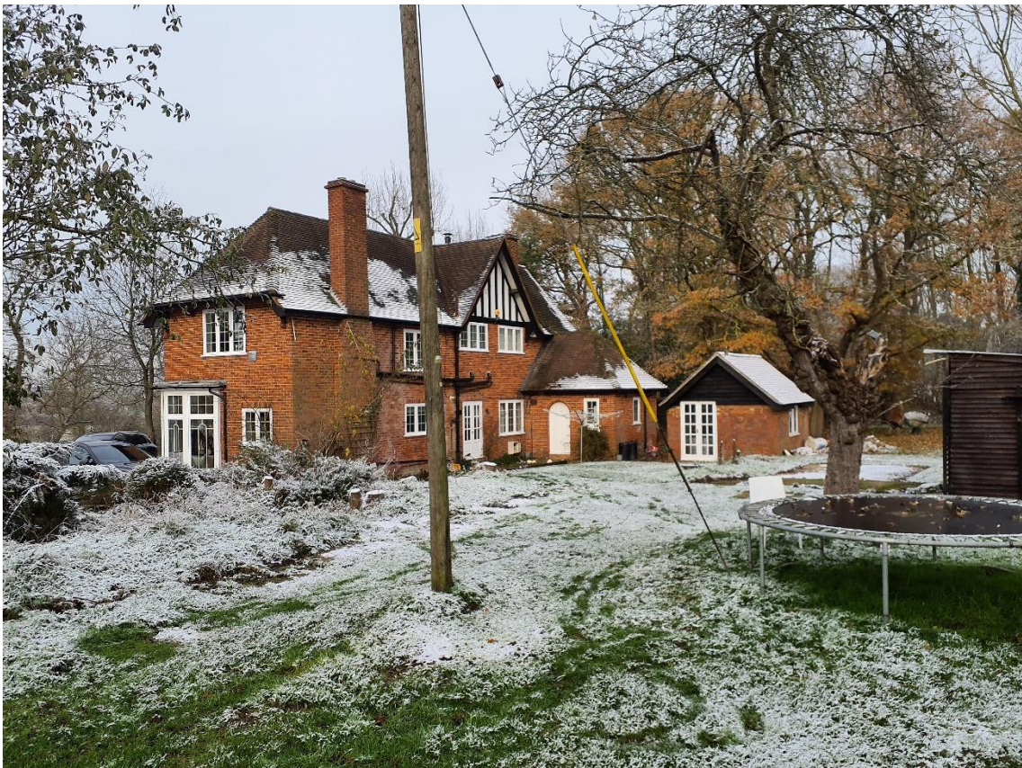
Figure 3 – Looking northwards at the existing dwelling and the area for proposed extension.
