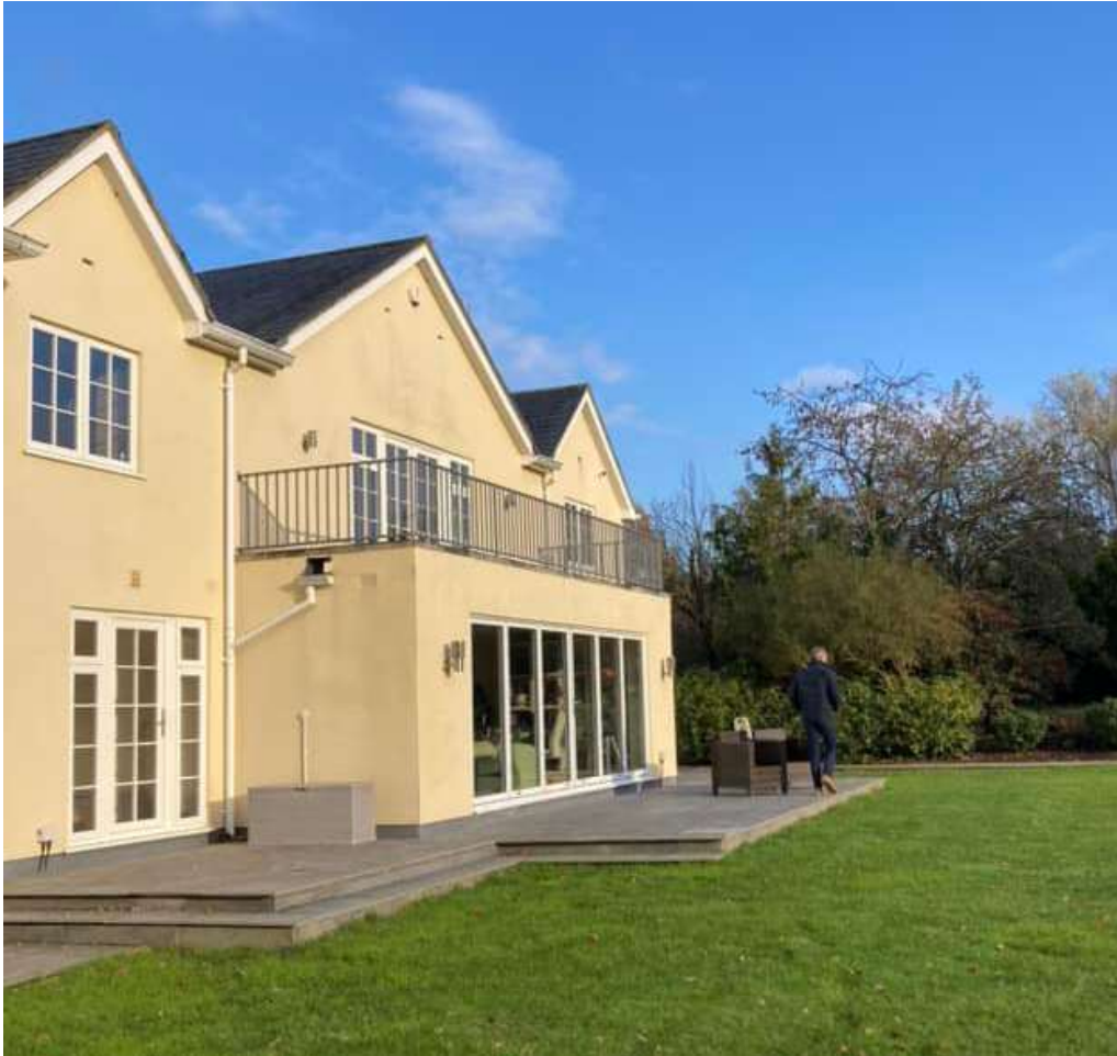
The south side of the existing house
