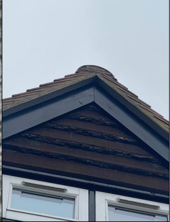
Photograph 18: Rear elevation wooden cladding.
