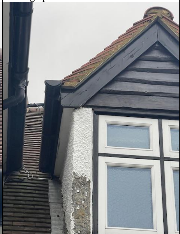
Photograph 8: Rear dormer windows with wooden cladding.
