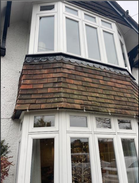
Photograph 22: Hanging wall tiles on the front elevation. Unaffected by works.
