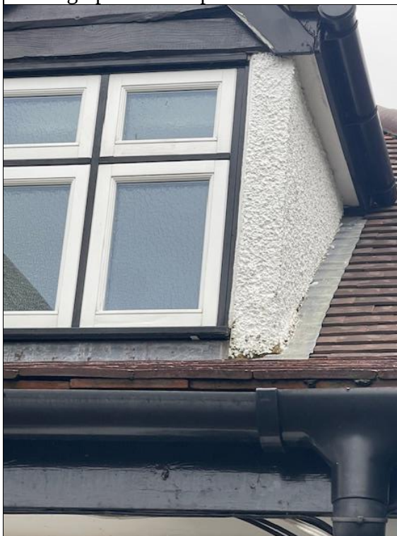
Photograph 7: Rear dormer windows with wooden cladding.
