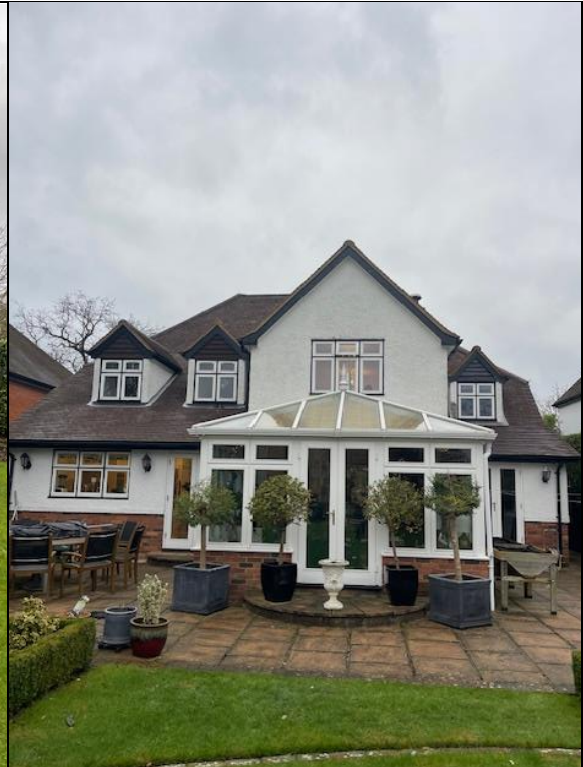
Photograph 10: Rear elevation with conservatory and patio.
