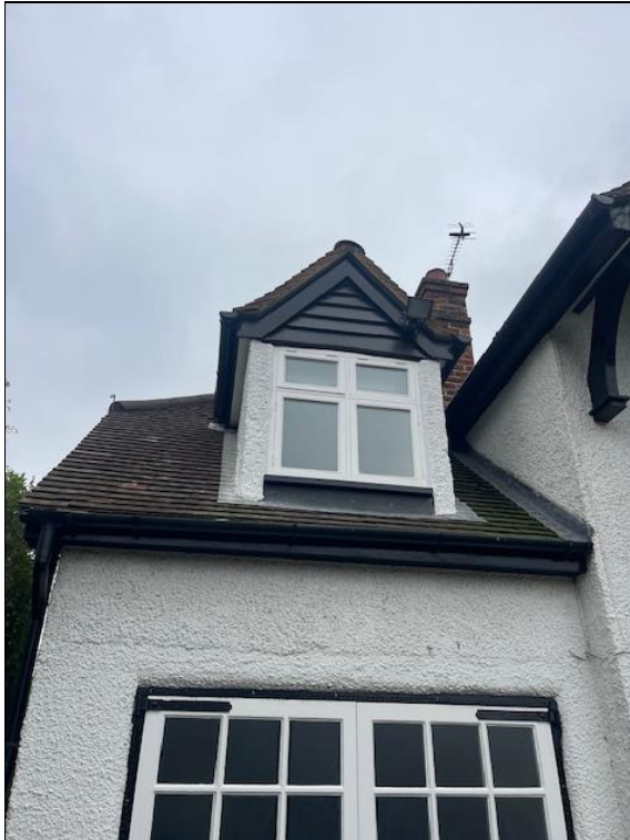
Photograph 21: Front elevation dormer window.
