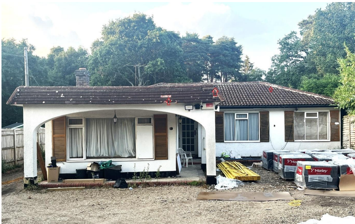
Figure 7. Front elevation of bungalow looking northeast: Red arrows indicate potential openings for crevice roosting bats.
