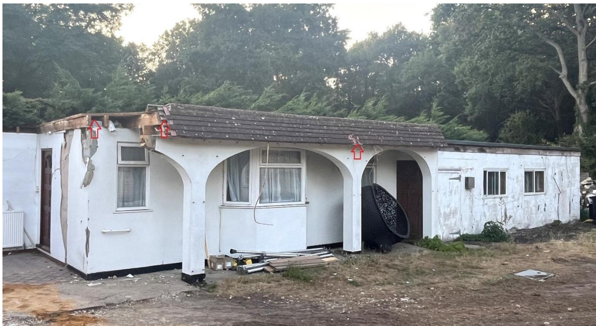
Figure 9. South face of rear extension looking north: Red arrows indicate potential openings for crevice roosting bats.
