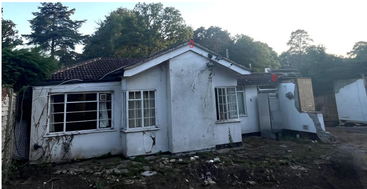
Figure 8. Rear elevation of bungalow looking southwest: Red arrows indicate potential openings for crevice roosting bats.
