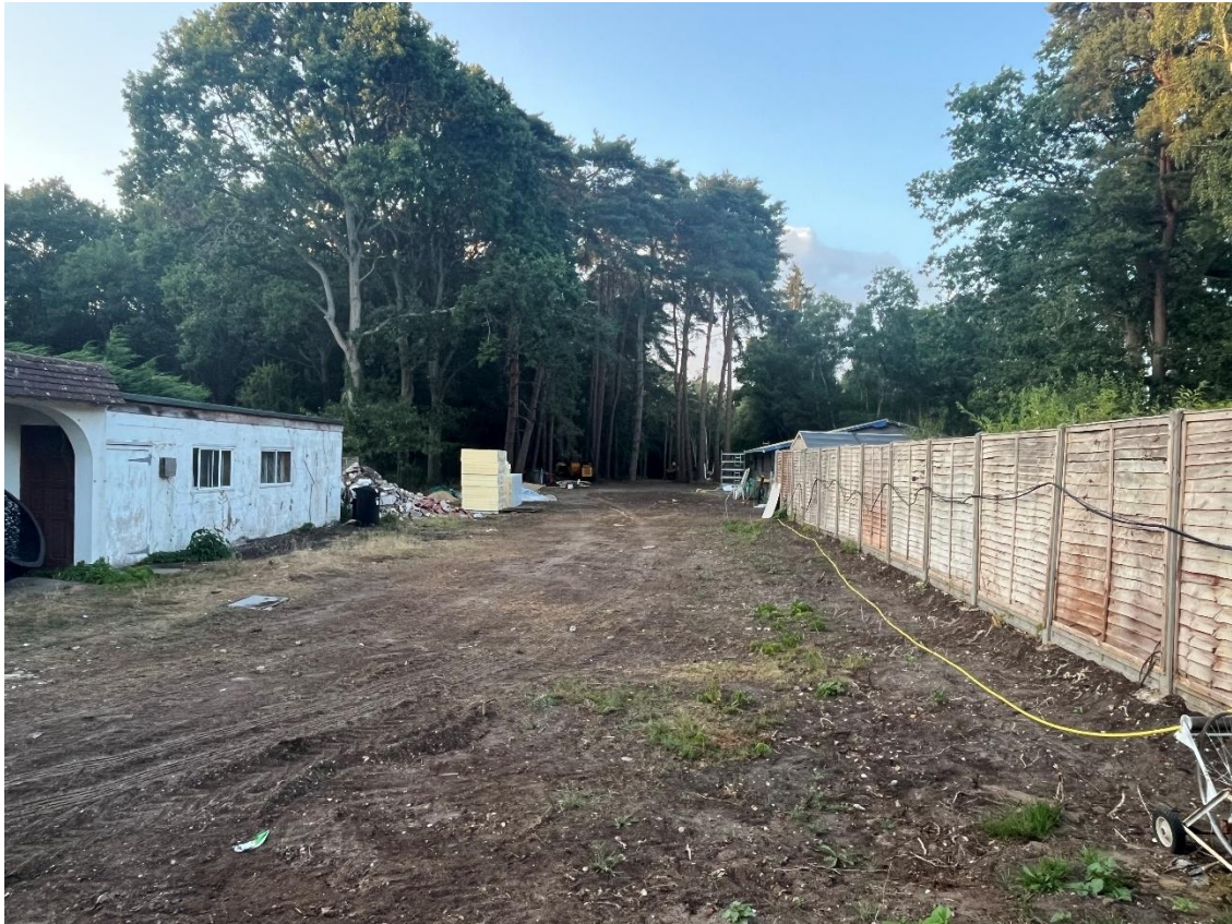
Figure 4. Looking northeast from back face of bungalow.
