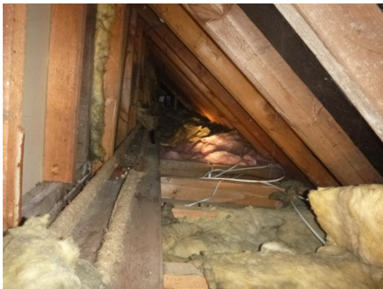
Photograph 15. Eaves void with fibreglass insulation.
