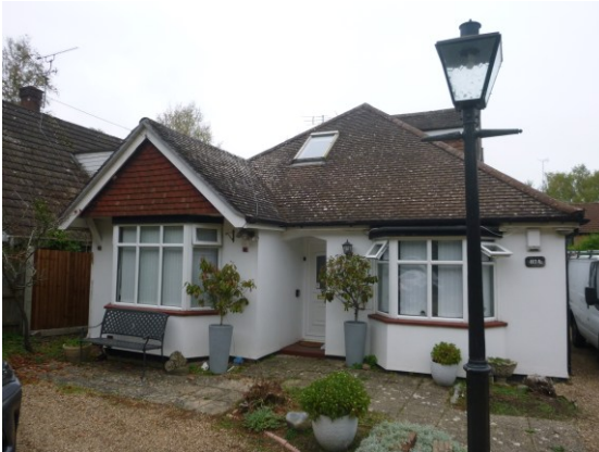
Photograph 1. Front of property viewed from south.
