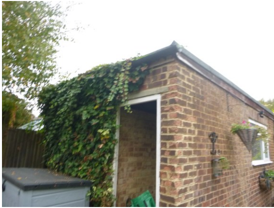
Photograph 13. Flat roof garage (TN10).
