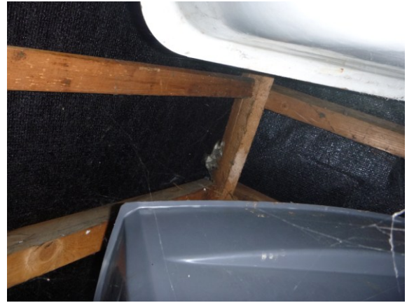
Photograph 26. Fully intact bitumen felt along the ridge.
