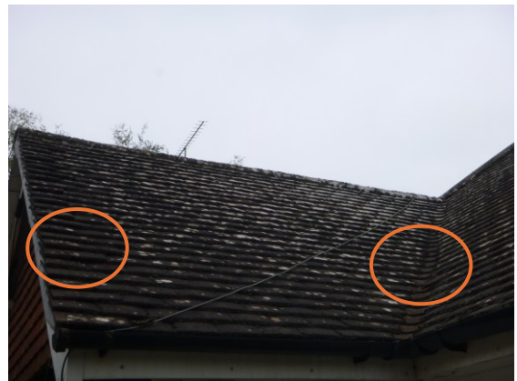
Photograph 4. Gaps under lifted verge tiles and in roof valleys ( TN3-4 ).
