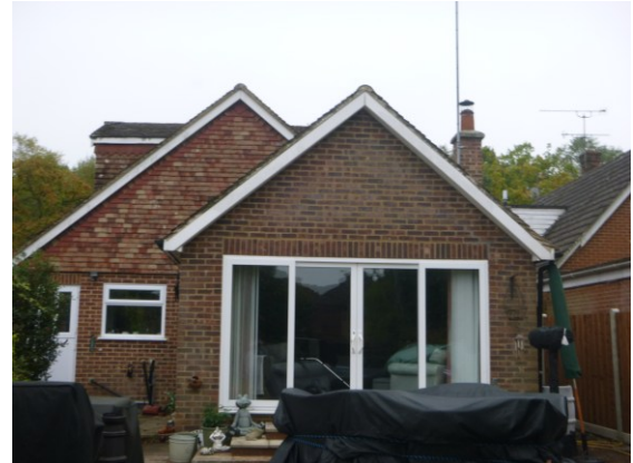
Photograph 2. Rear of property viewed from north.
