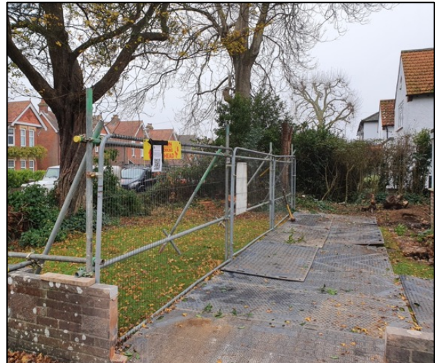
GP2: Tree protection barriers & trackmat ground protection
