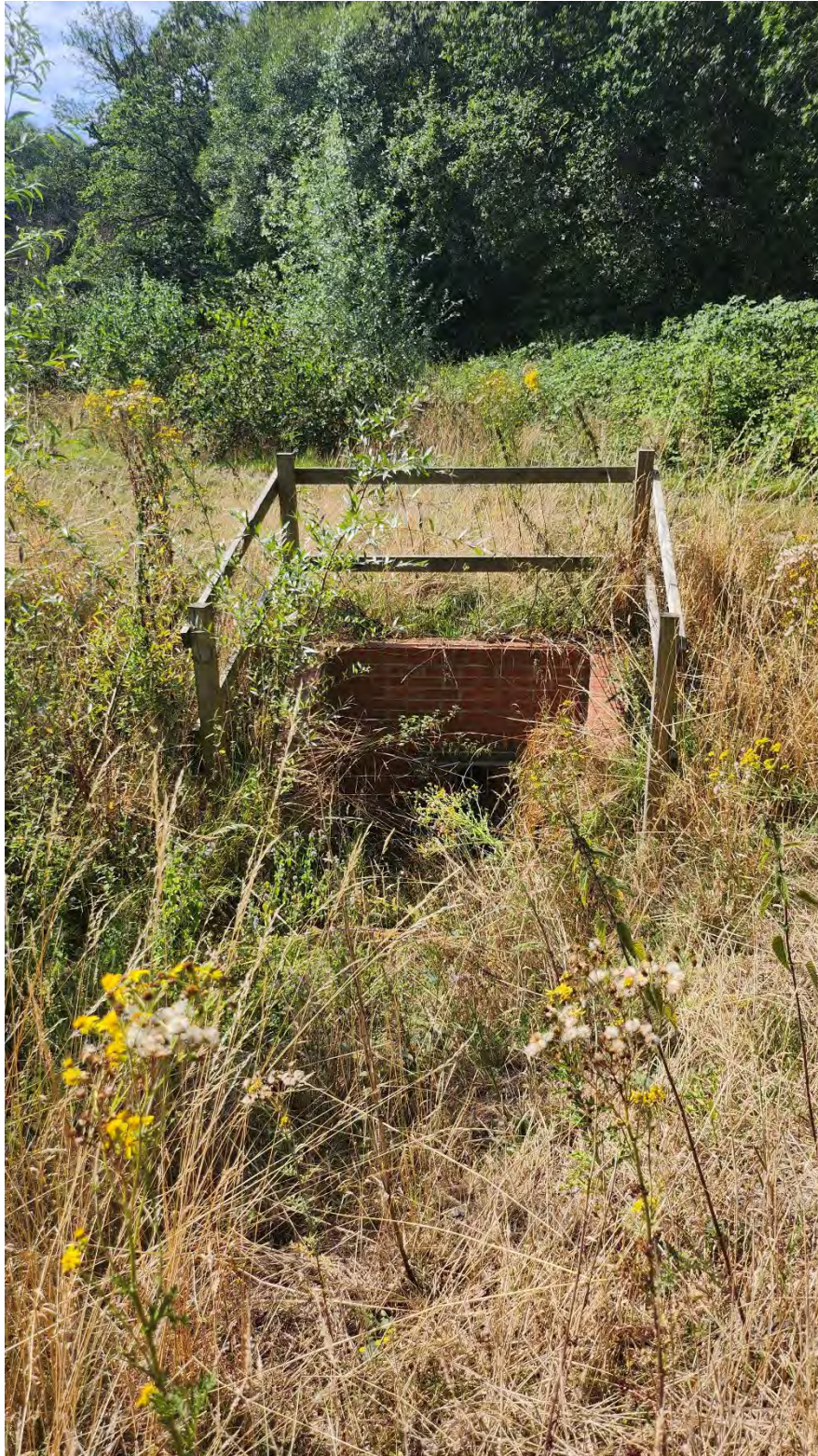
Plate 16 View of culverted waterway located in the north western corner of the western field
