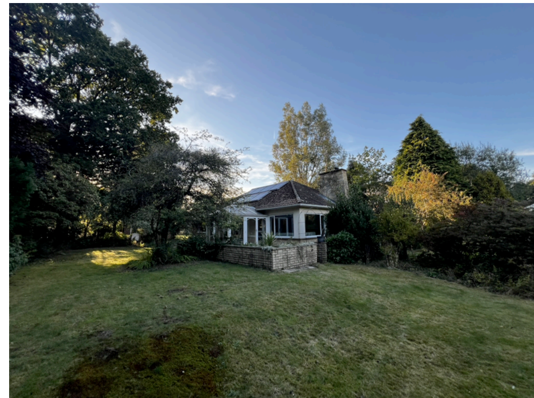
Plate 8 View looking west from the garden of No 121 NGL showing the rear/side elevations of the existing dwelling with the mature, perimeter planting/screening the plot.
