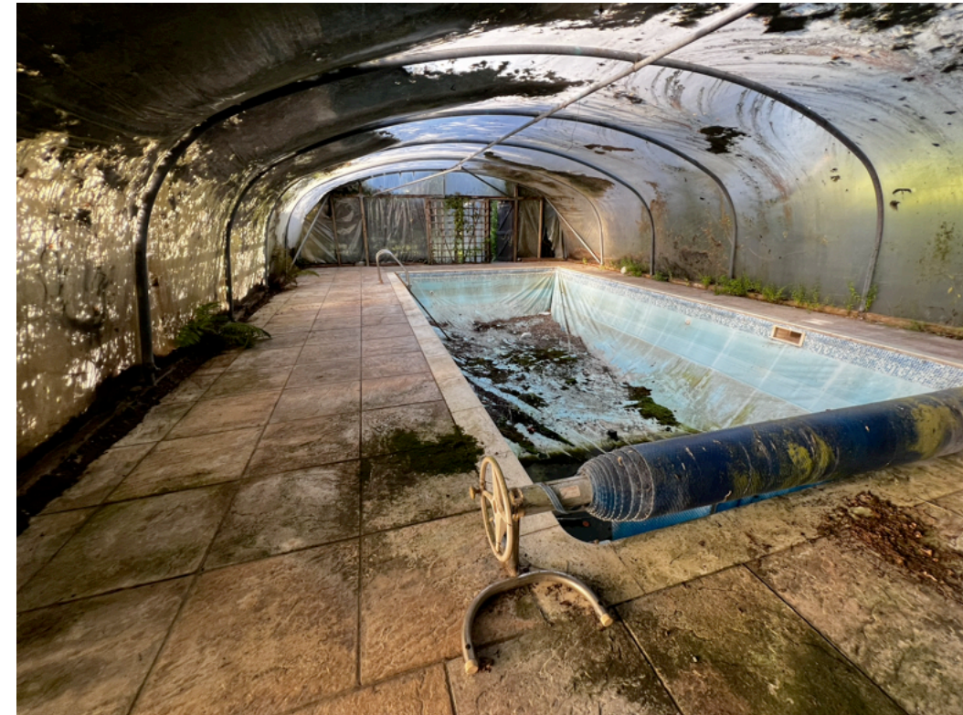
Plate 10 Existing swimming pool and enclosure. Enclosure to be demolished and pool infilled and landscaped.
