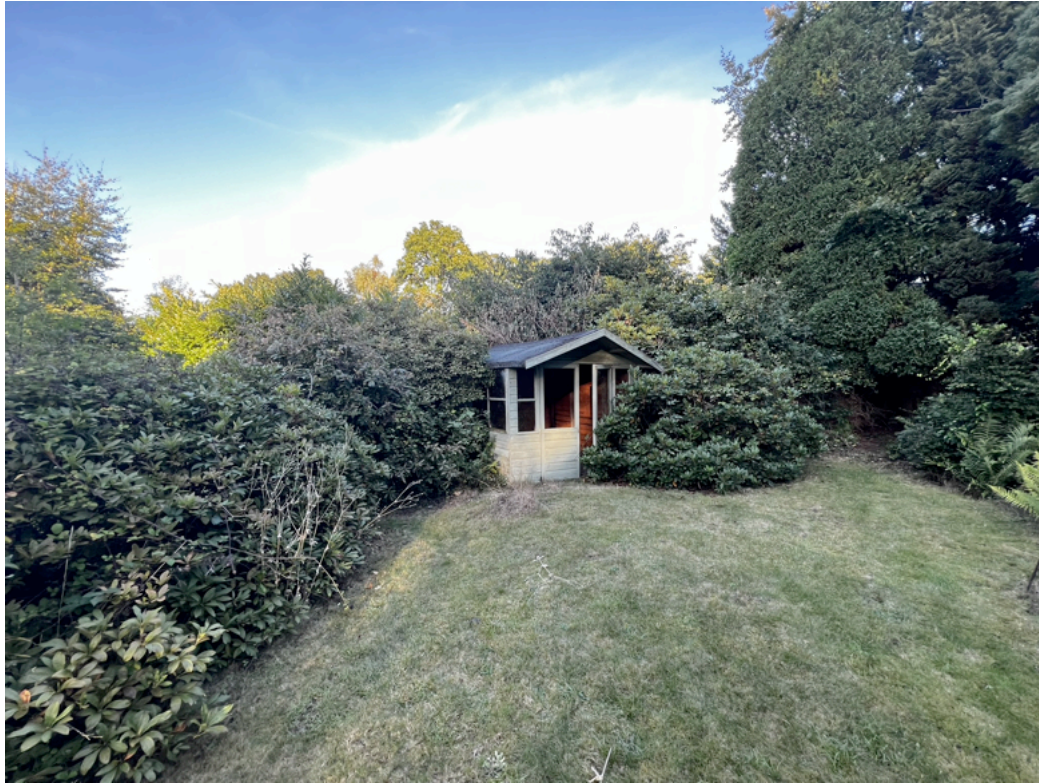
Plate 9 Existing Summerhouse to be demolished.
