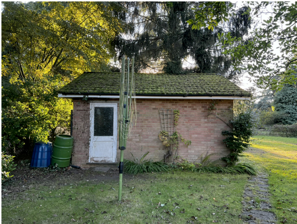
Plate 11 View showing side elevation of detached double garage to be demolished.
