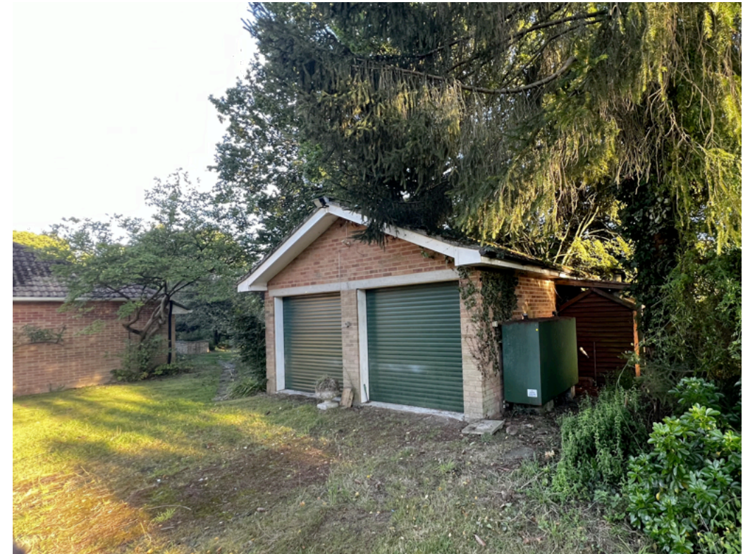
Plate 12 View showing detached double garage to be demolished.
