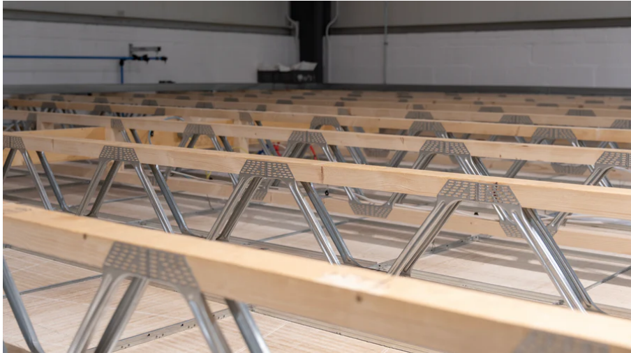
Open webbed metal/timber joist system
