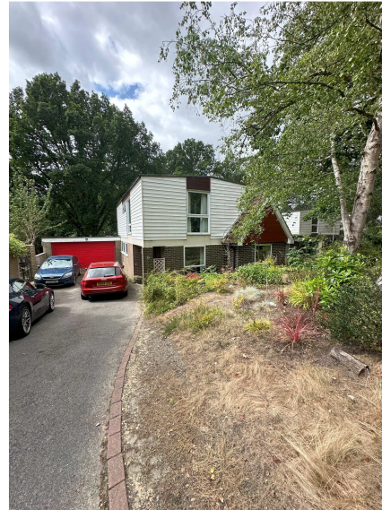
View from Driveway
