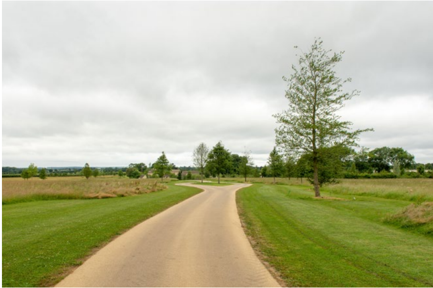
Full depth coloured asphalt Colour: Buff Accessories: 6mm metal edging Vehicular loaded
