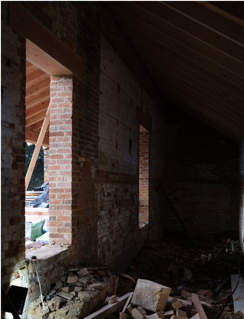
Photo 2: Internal view of the former window location, showing the resultant reduction in natural daylight.
