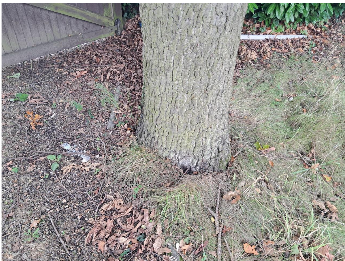
Photo 3 – Driveway kinks around the base of T006 (Oak)
