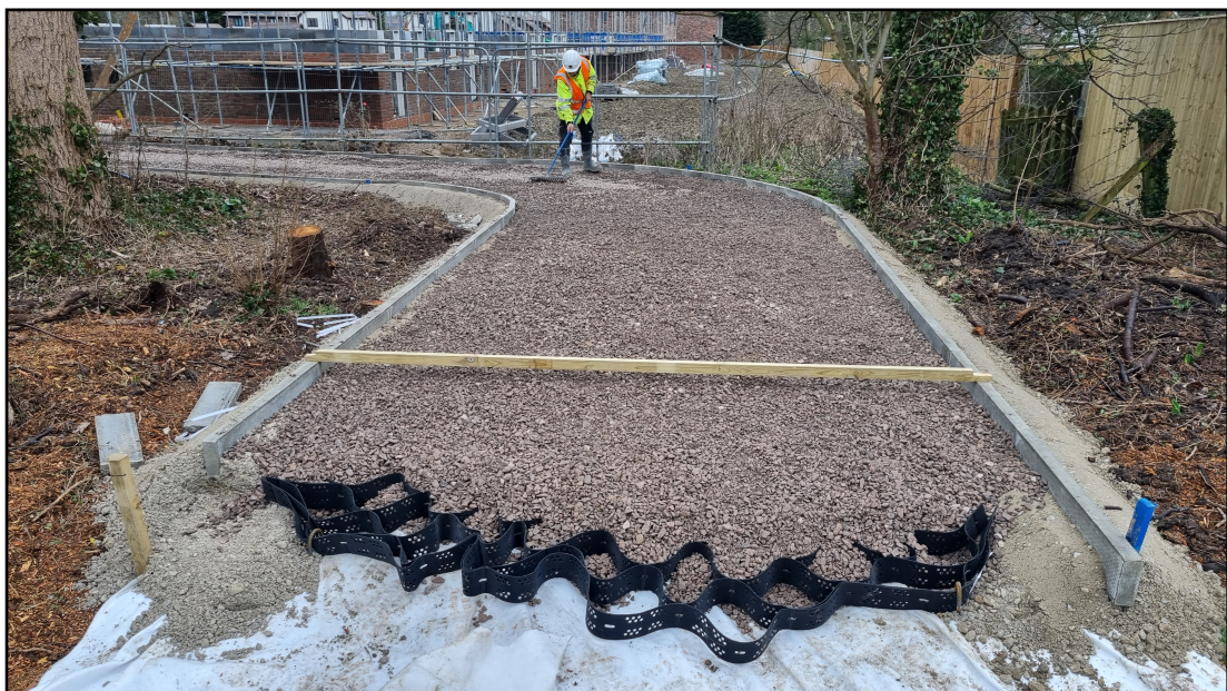
ND2: Example of no-dig surface installation
