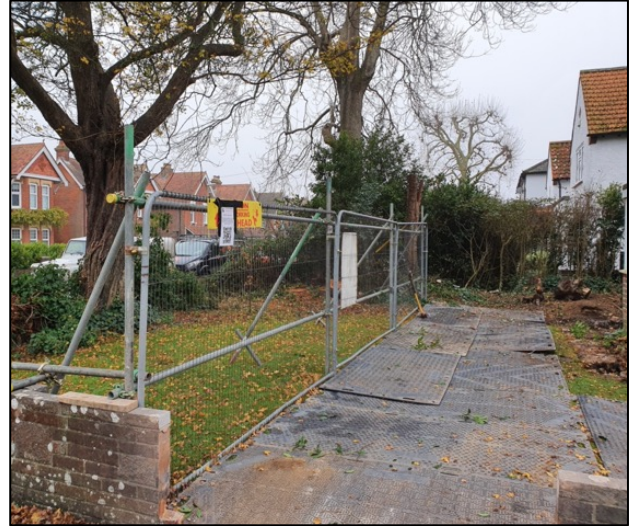
GP2: Tree protection barriers & trackmat ground protection
