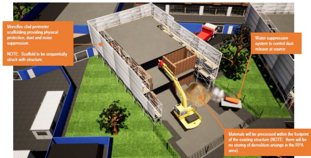
Example of open face demolition
