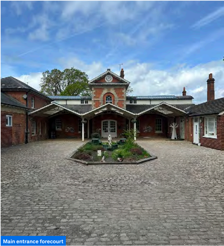
Main entrance forecourt
