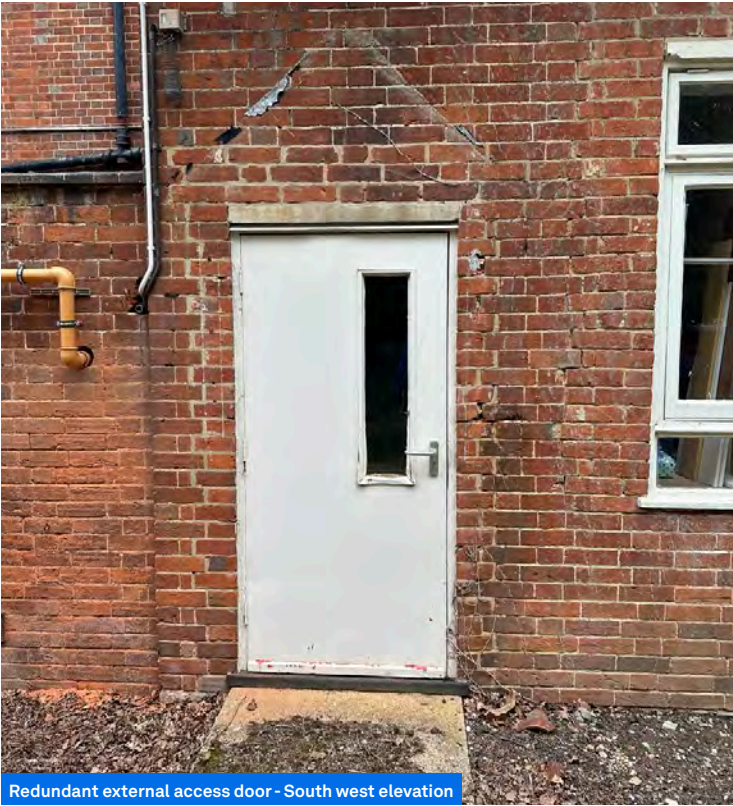
Redundant external access door - South west elevation
