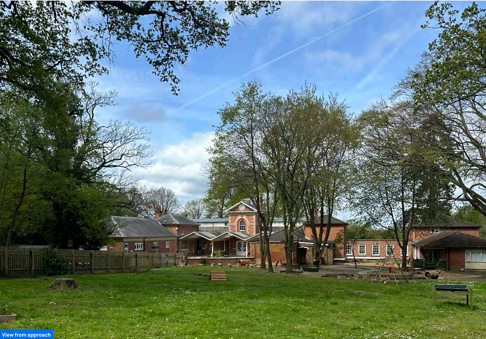
View from approach
