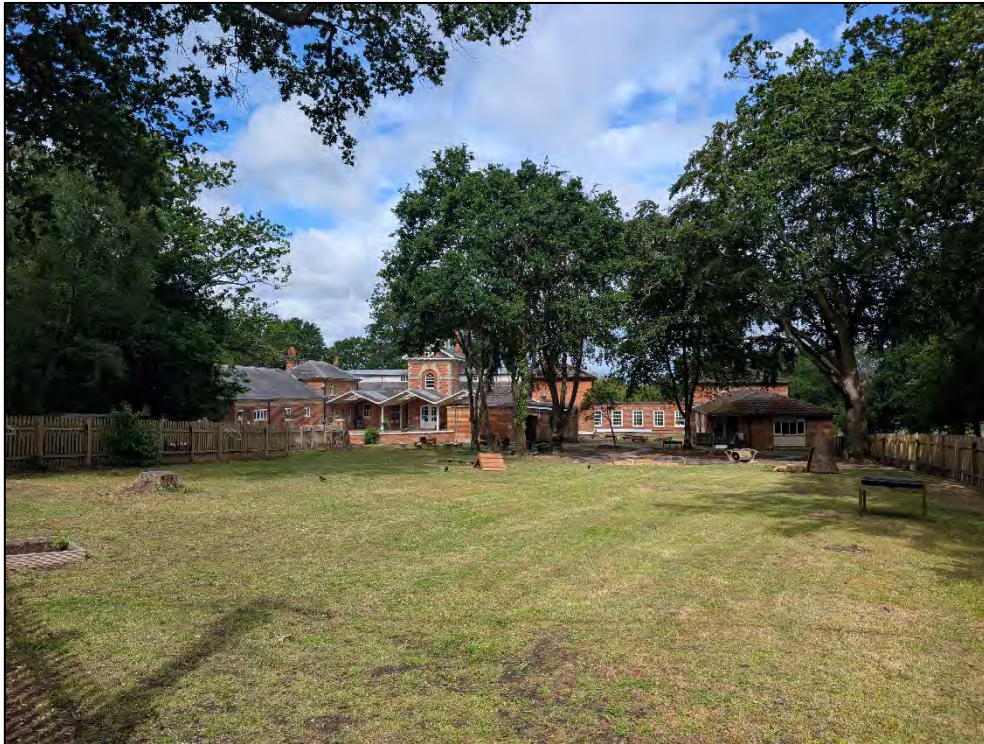
Plate 1 The Early Learning School, formerly the Stables and Coachman's House. Viewed from east
