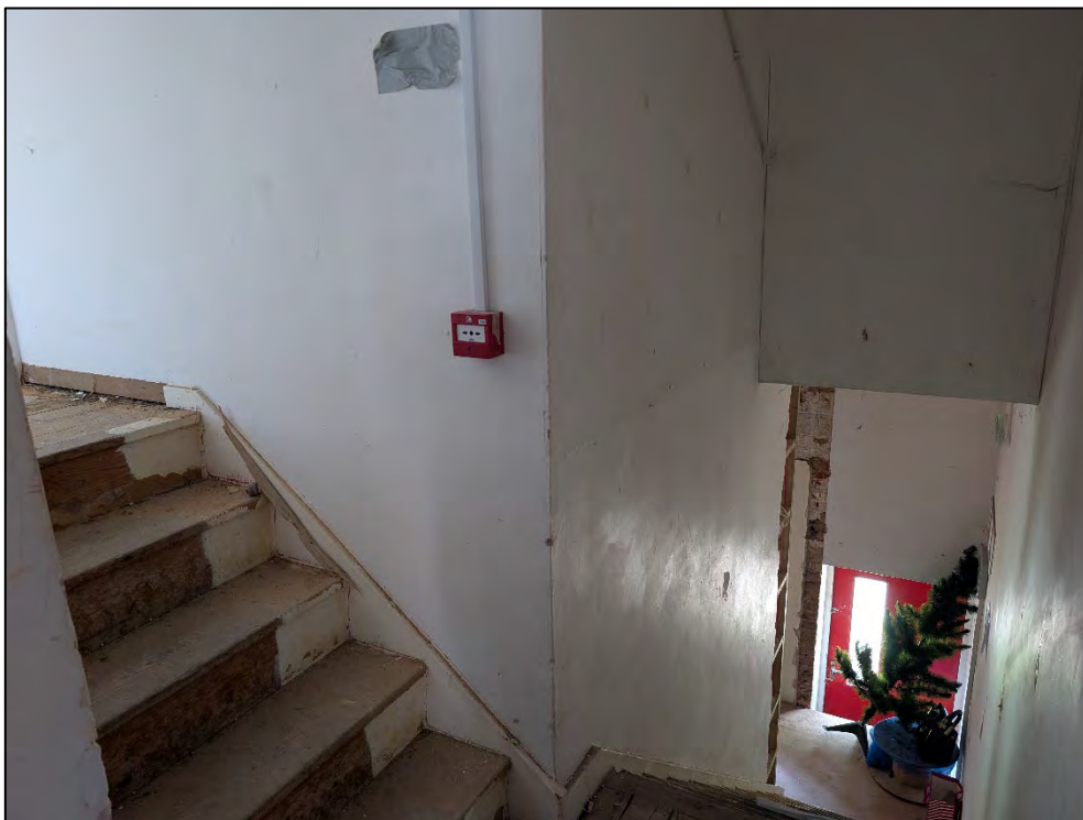
Plate 4 West Wing internal staircase arrangement. Viewed from north
