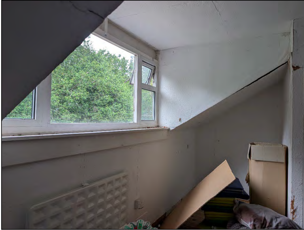
Plate 5 West Wing internal room arrangement. Note modern uPVC windows, radiator fixing and electrical sockets
