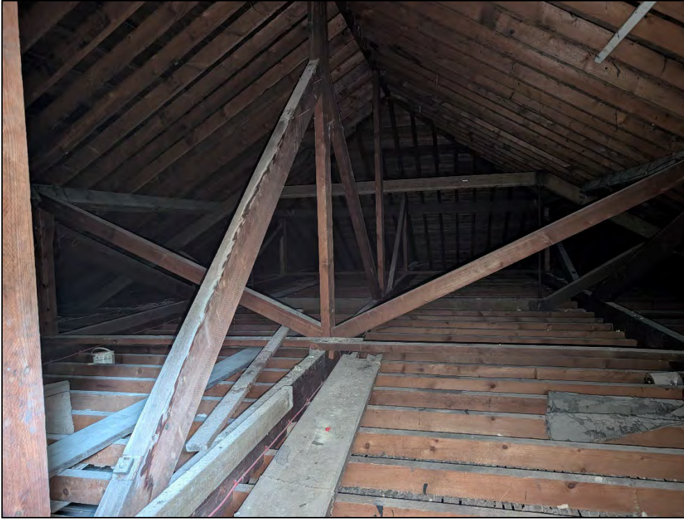
Plate 11 West Wing internal room arrangement. Note internal sawn timber roof structure
