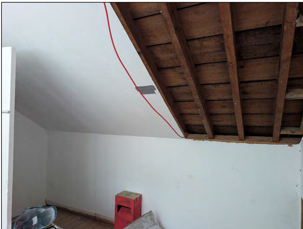
Plate 10 West Wing internal room arrangement. Note exposed timber roof structure
