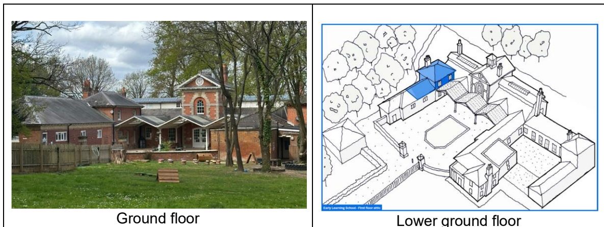
Figure 2: General photograph and illustrative view of attic area
